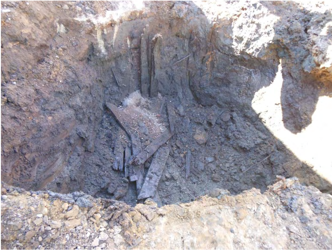
Photo 3. UST Excavation Approximately 8 feet bgs
