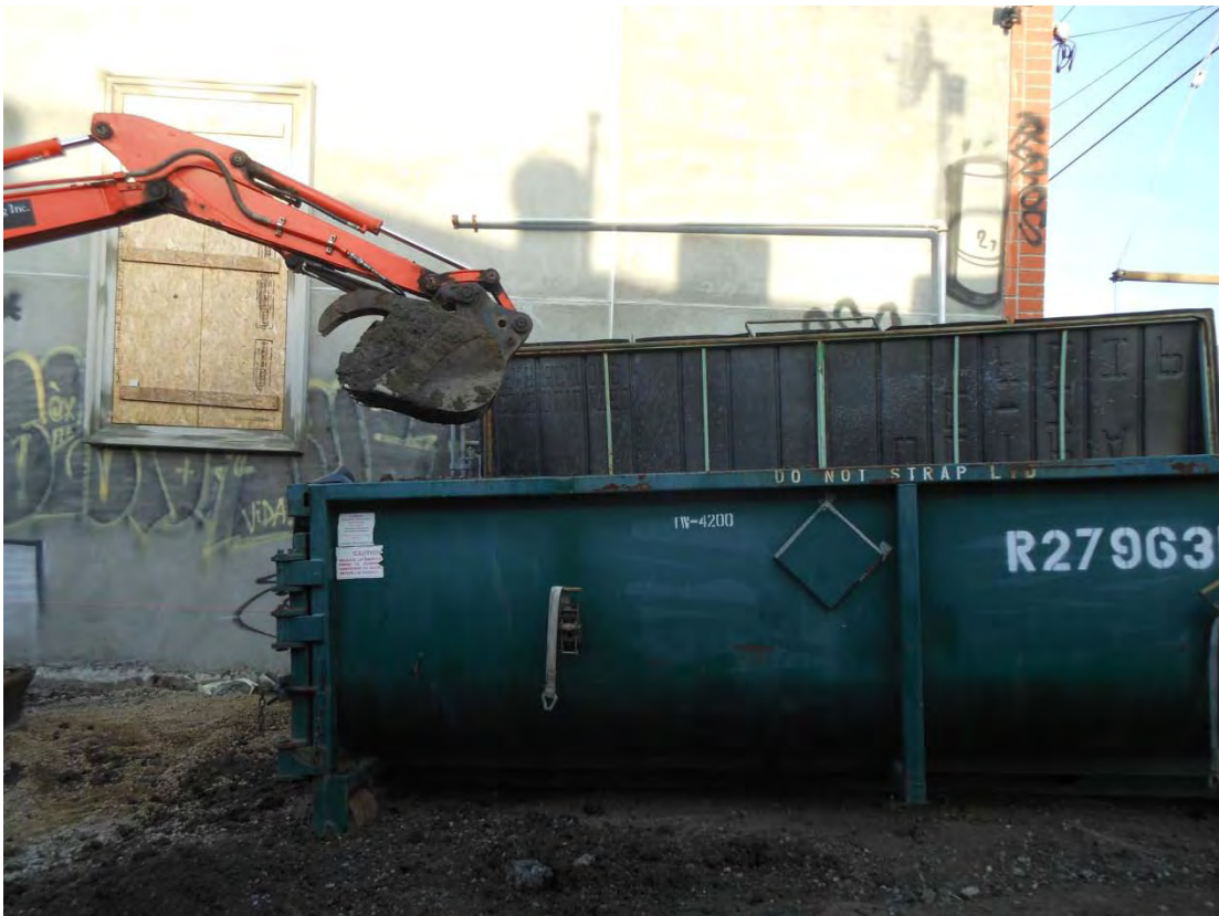
Photo 4 Loading Contaminated Soil into Roll-Off Bin
