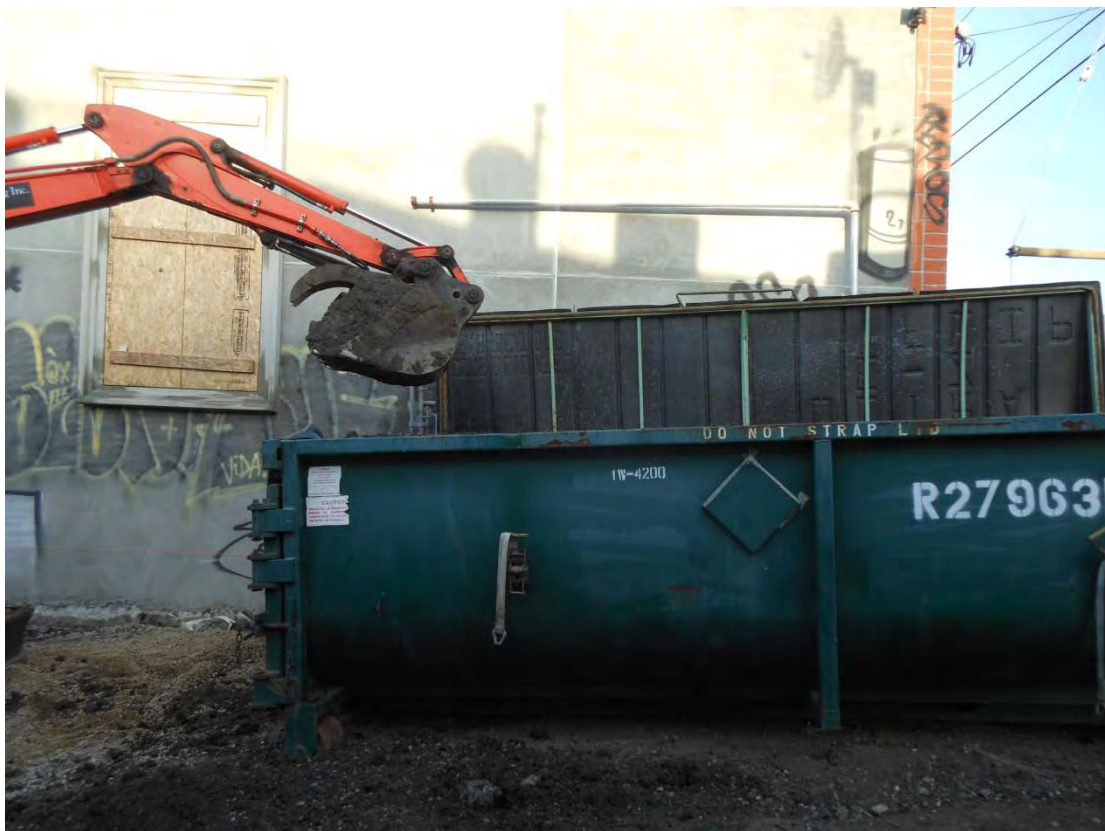
Photo 4 Loading Contaminated Soil into Roll-Off Bin
