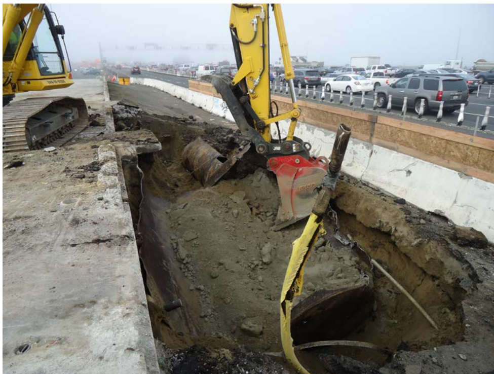
Photo 16 – View of sand slurry in UST #3 being excavated prior to removing tank from the ground.
