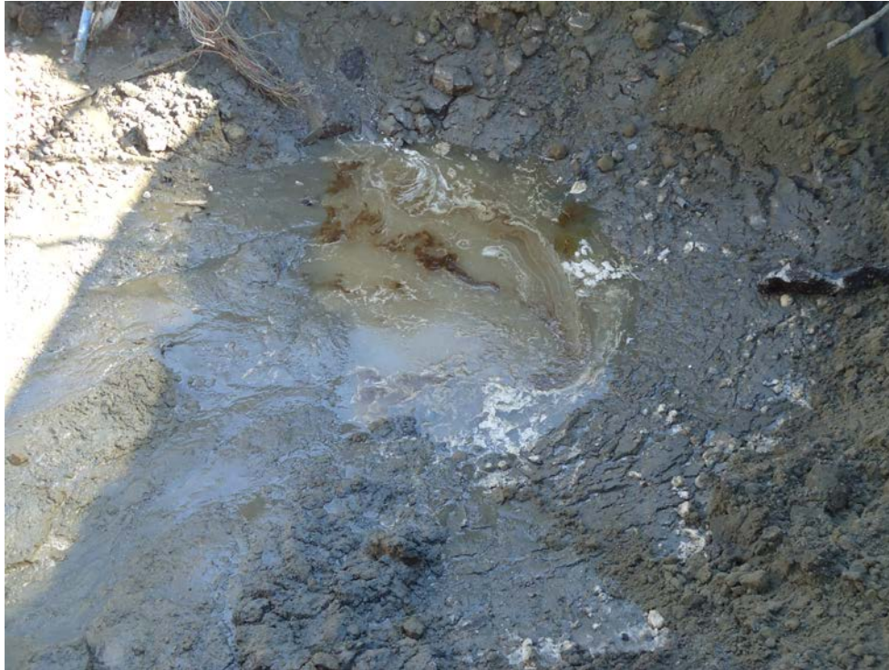
Photo 19 – View of free product remaining in UST #1 excavation after groundwater had been removed.
