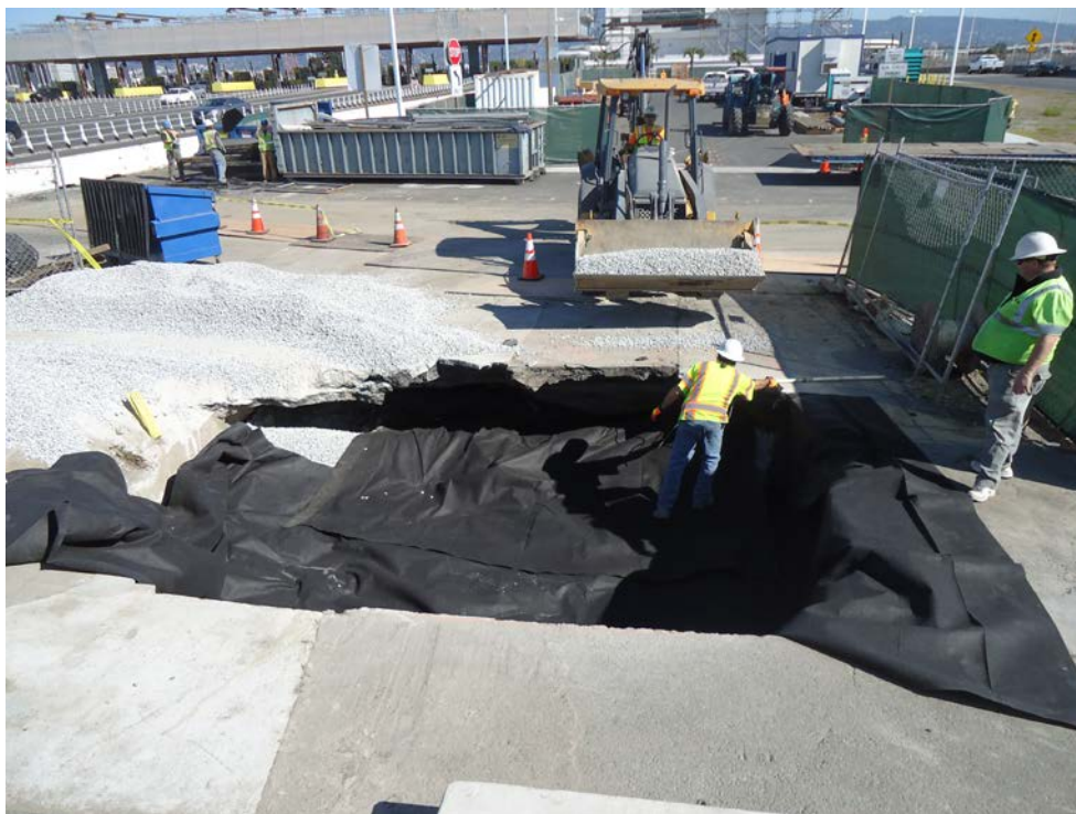
Photo 8 – View of filter fabric being placed in UST #1 excavation during backfilling operations.
