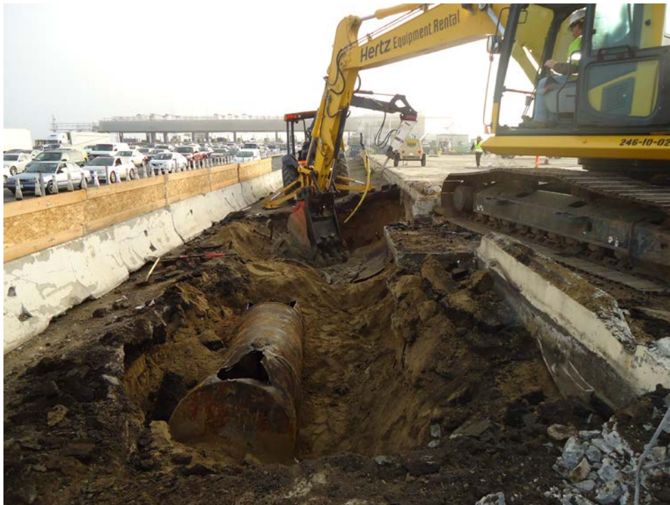
Photo 10 – View of the top of UST #2 after the ends of the tank were further opened using a rivet buster.
