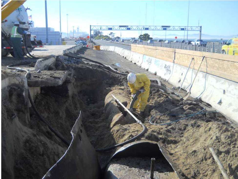
Photo 9 – View of fuel oil being removed from UST #2.
