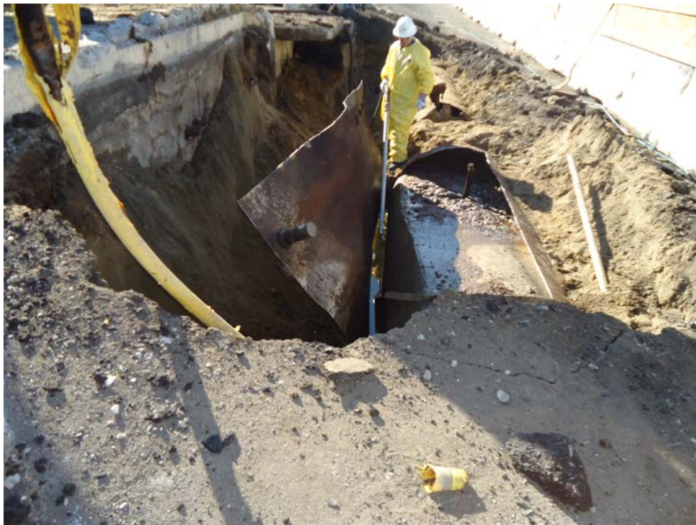
Photo 14 – View of residual fluids in UST #3 being removed by NRC.
