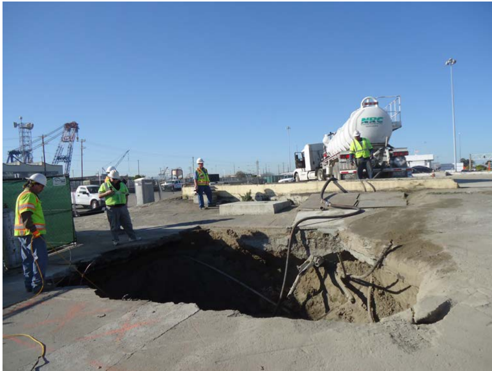
Photo 7 – View of NRC removing petroleum hydrocarbon-impacted groundwater from UST #1 excavation.
