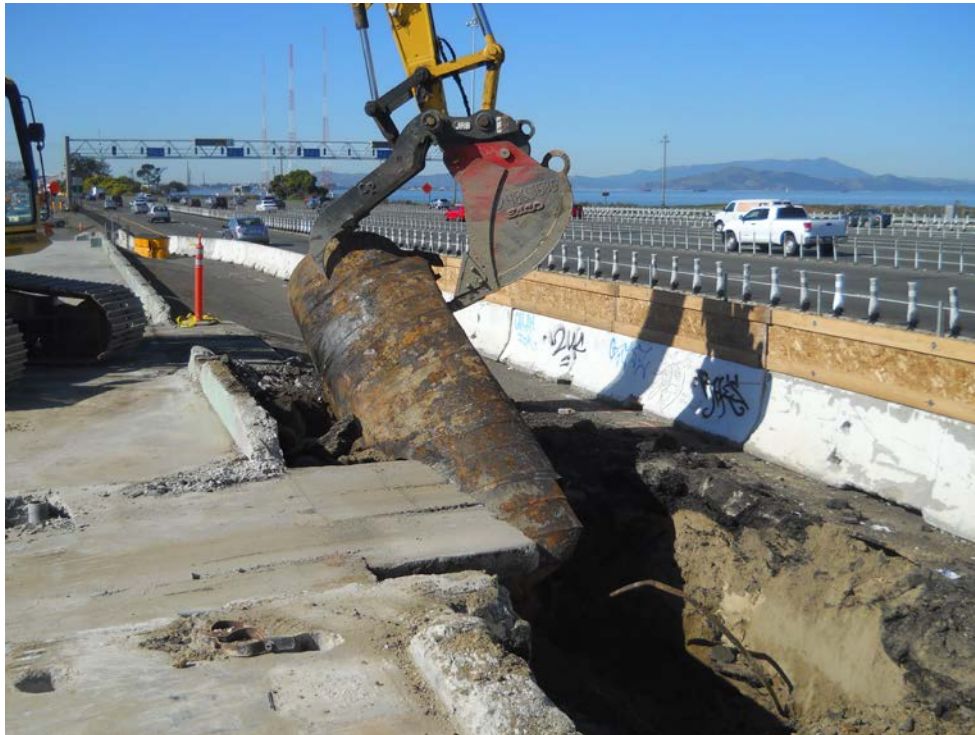
Photo 11 – View of UST #2 being removed from excavation.
