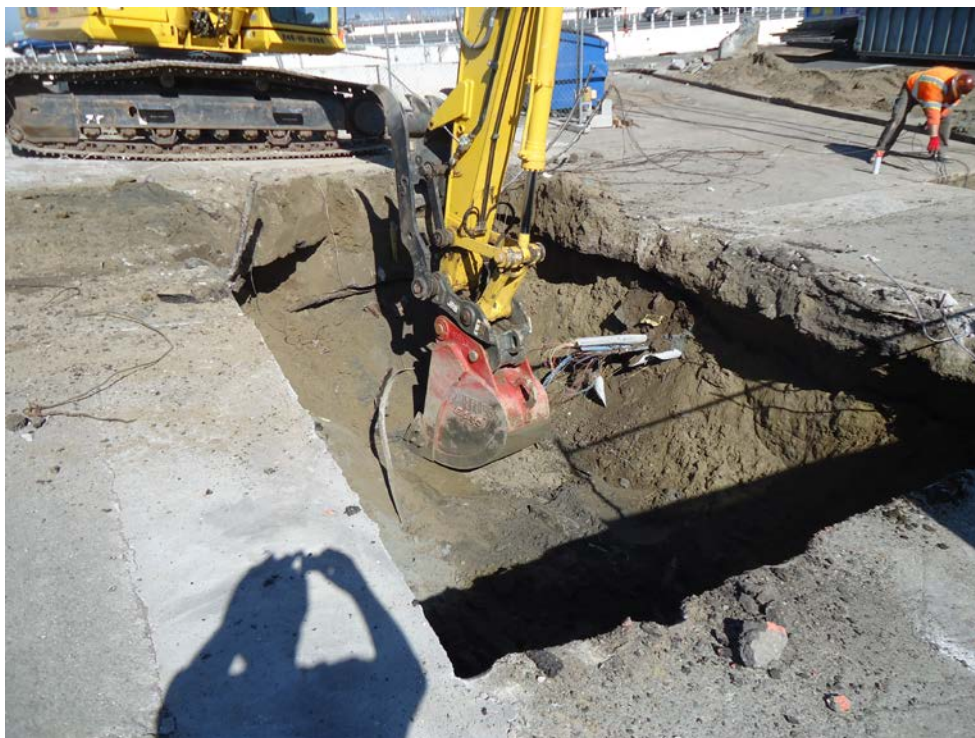
Photo 2 – View looking northeast as UST #1 as the top of the UST is being unearthed.
