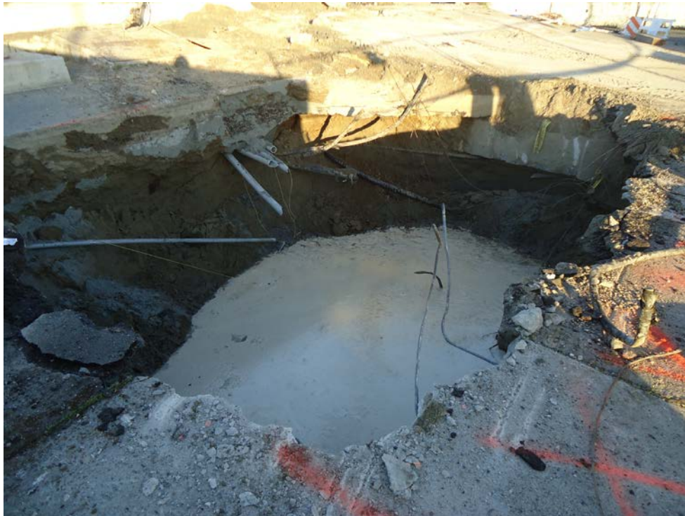
Photo 5 – View looking at UST #1 after UST was removed and groundwater entered the excavation.
