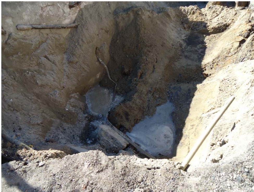
Photo 20 – View of groundwater in east end of UST #2/UST #3 excavation beneath UST #3.
