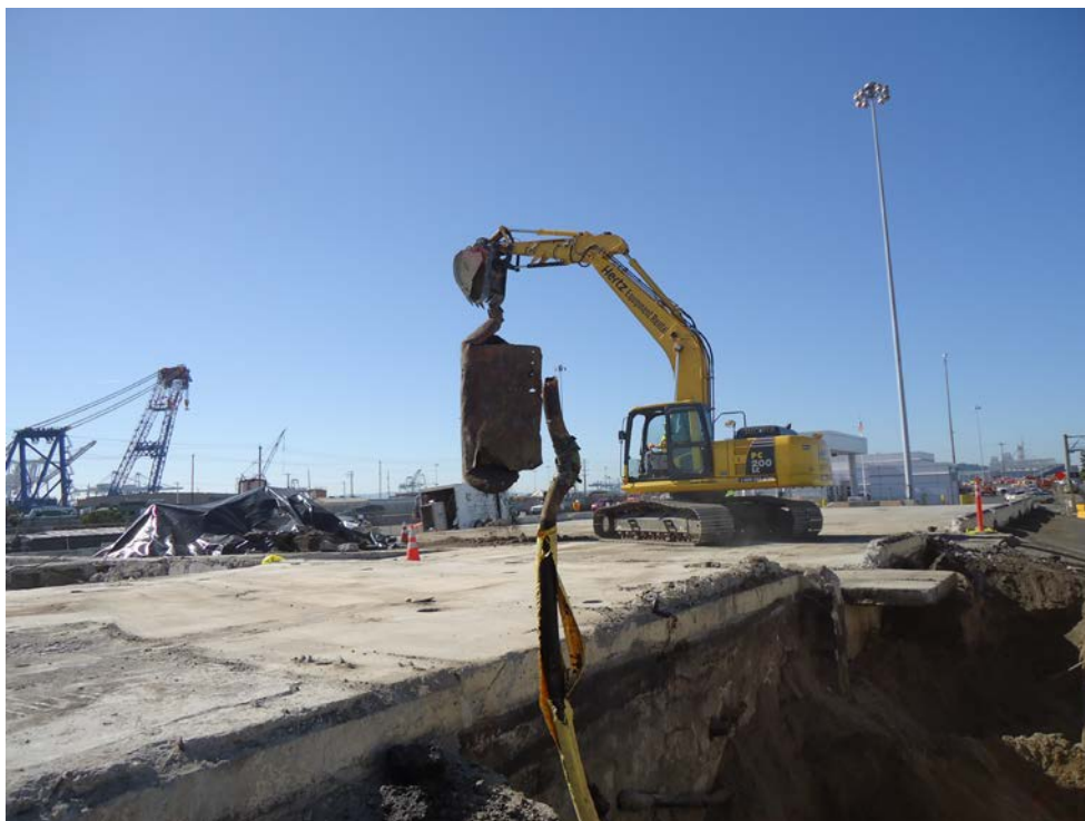
Photo 18 – View of UST #3 being further emptied of sand slurry prior to being crushed.
