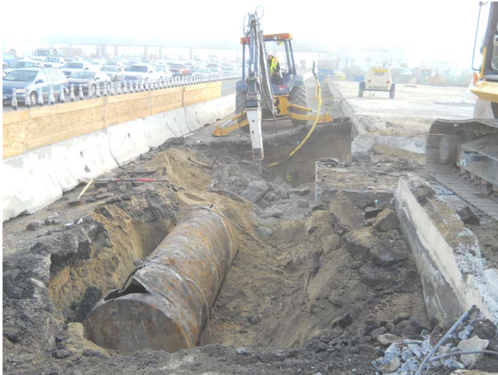
Photo 15 – View of sand slurry in UST #3 being broken up pneumatic hammer.
