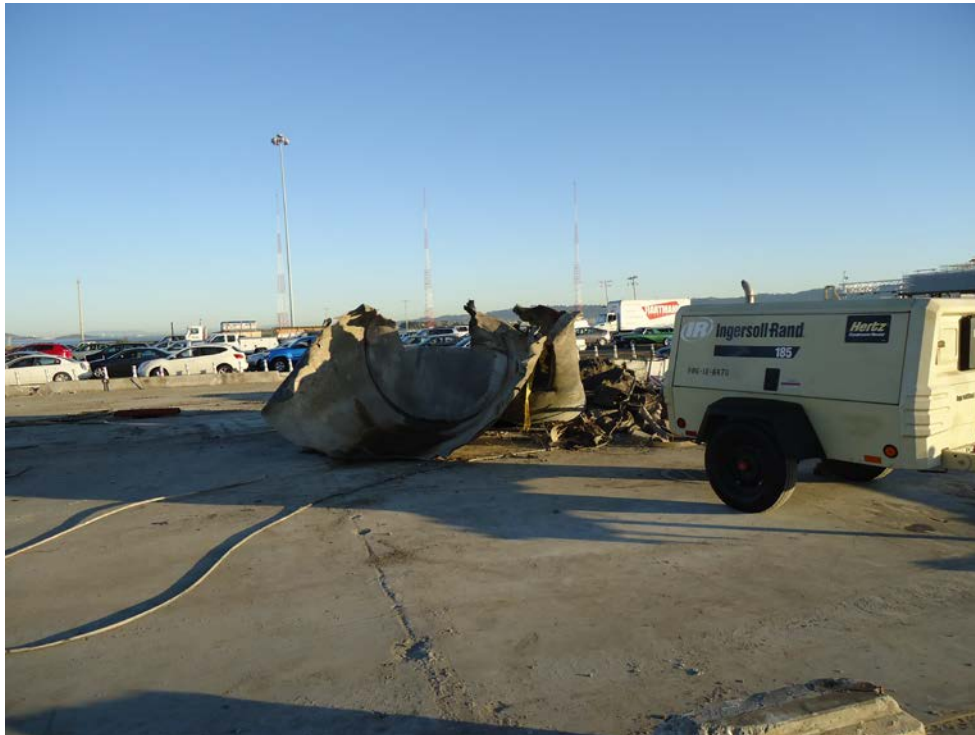
Photo 3 – View of UST #1 after top was torn open and sand slurry was removed from the tank.
