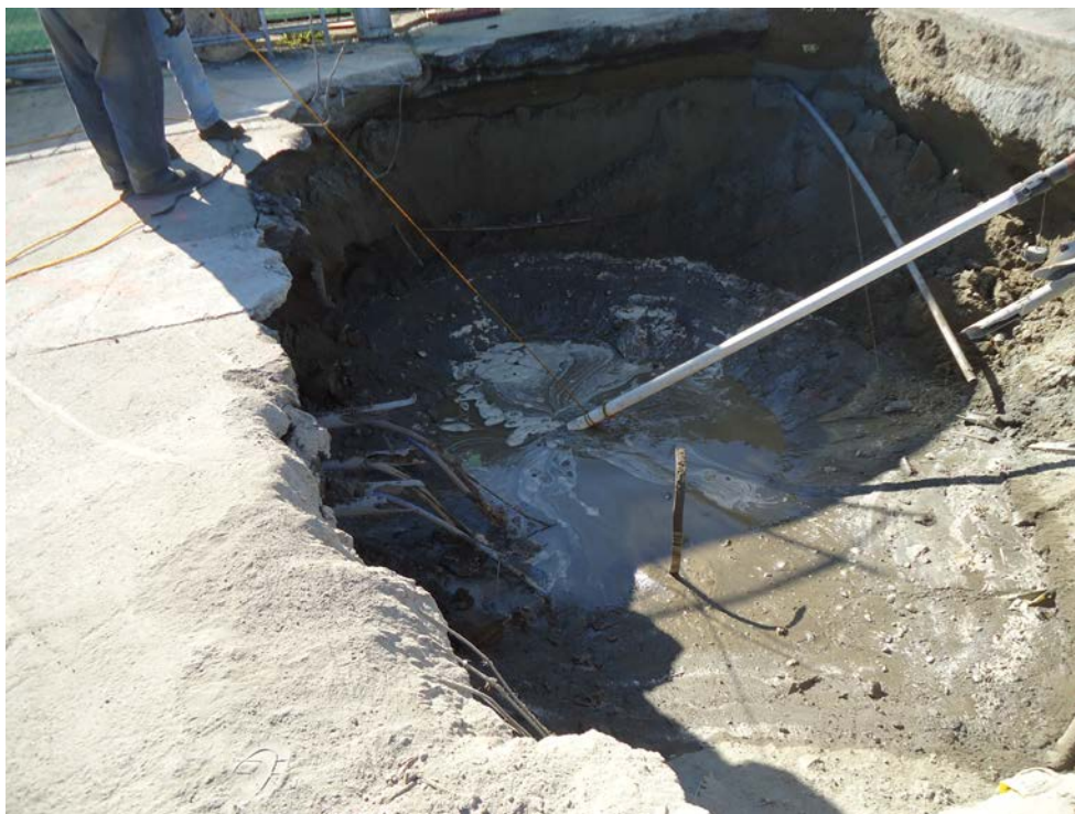
Photo 6 – View of petroleum-impacted groundwater in UST #1 excavation being removed prior to backfilling.
