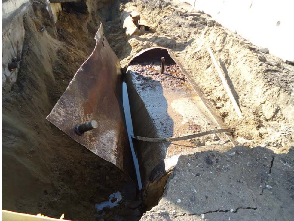
Photo 13 – View of UST #3 after the top was peeled back and the sand slurry inside tank was exposed.
