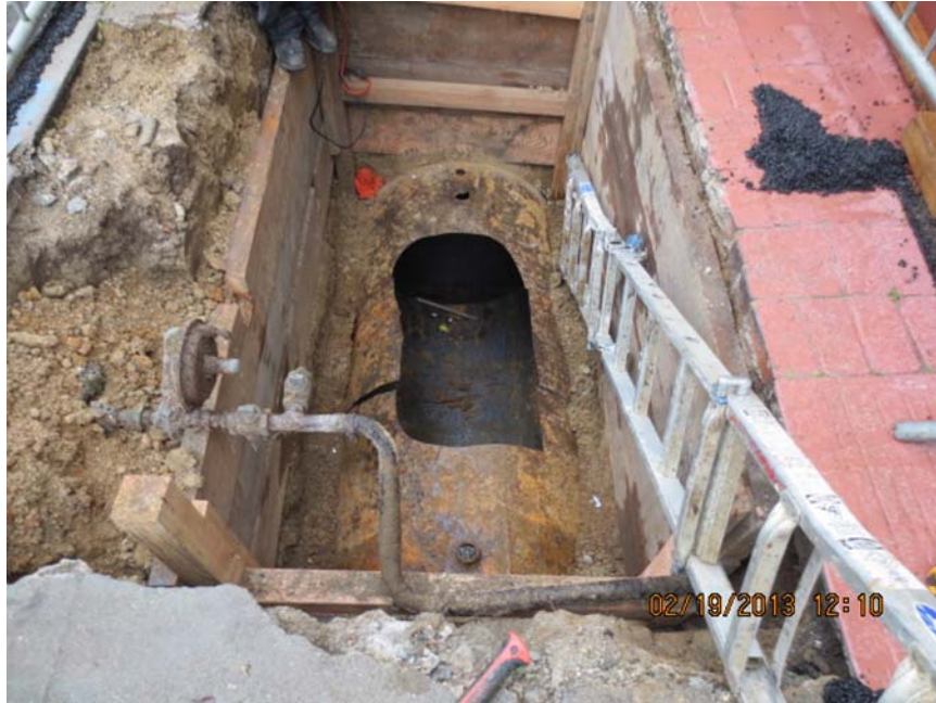
UST READY TO BE REMOVED FROM EXCAVATION
