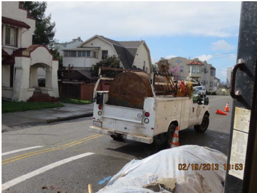
TANK READY TO BE TRANSPORTED FOR DISPOSAL
