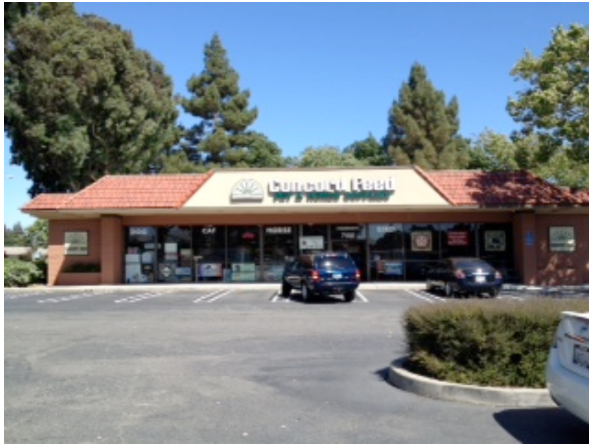
Photo 5: One-Story Commercial Building (Facing East) Located on Eastern Portion of Site
