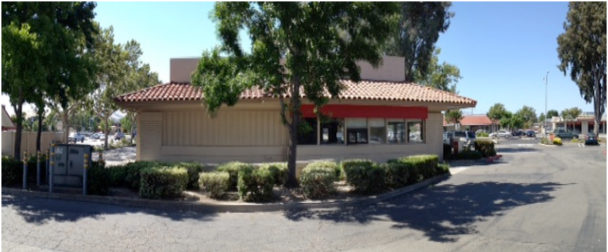
Photo 2: One-Story Commercial Building (Facing Northwest) Exterior of Western Building on Subject Site
