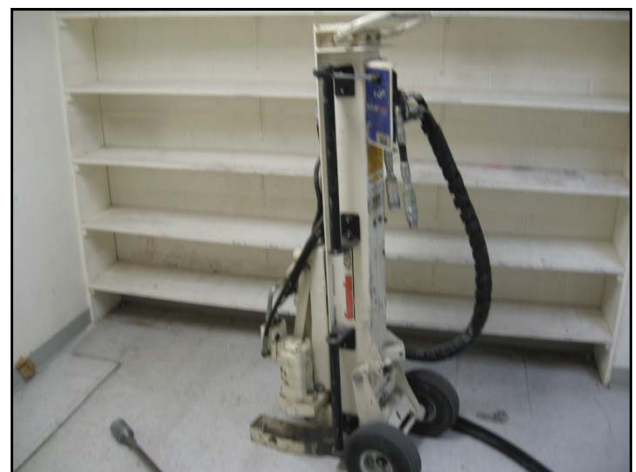
Photograph 12: A dolly-mounted, limited-space Geoprobe rig was used to drill boring B2.
