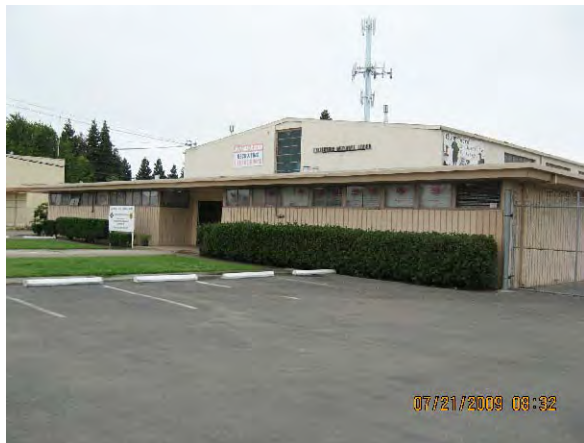
PHOTOGRAPH 1. Overview of site from northeastern boundary, shows armory building in foreground and adjacent cellular tower in background.
