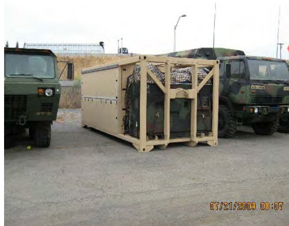
PHOTOGRAPH 6. Water purification with installed diesel generator. Generator was unused and had not previously been fueled.
