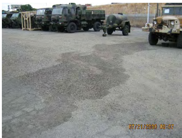
PHOTOGRAPH 3. Surface staining at northwest corner of armory building.
