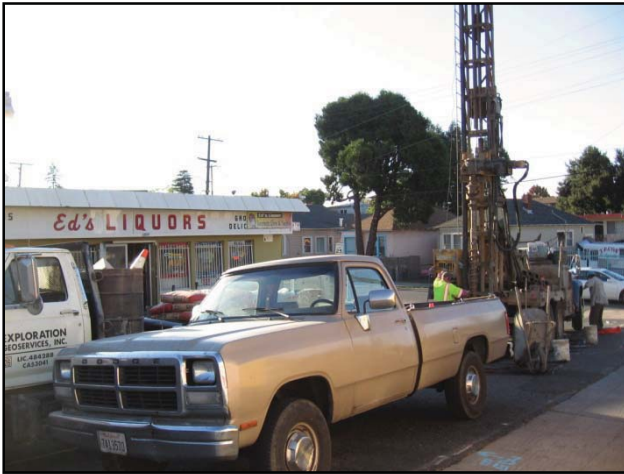
Photograph 1: The monitoring wells were installed using a 6-inch-diameter, hollow-stem auger rig.
