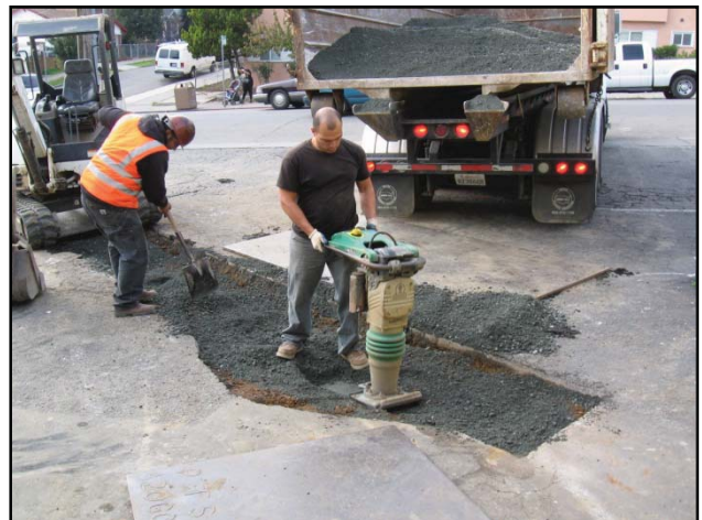
Photograph 6: The imported fill material was compacted using jumping jacks.
