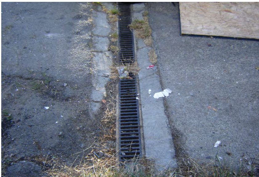
6. A picture of a trench drain located on the subject property.
