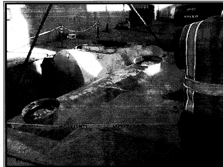
Photos 1 & 2: USTs immediately prior to extraction from UST pit
