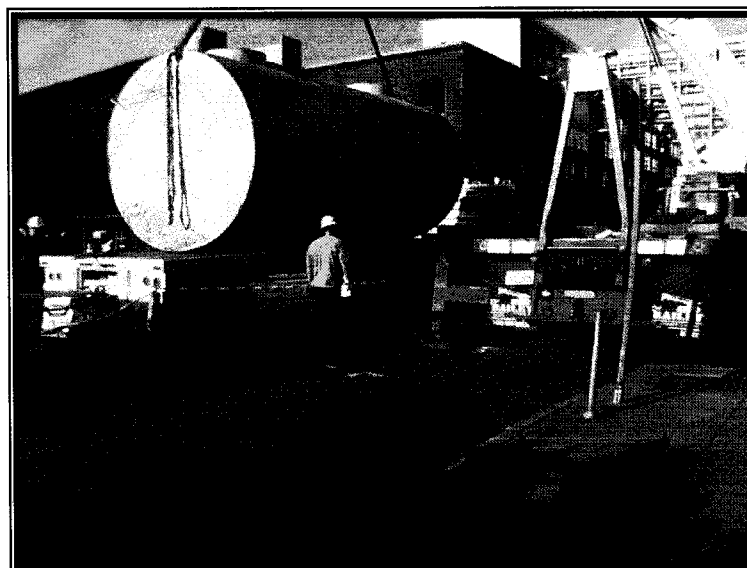
Photo 3: 10,000-gal UST hoisted on to flatbed.
