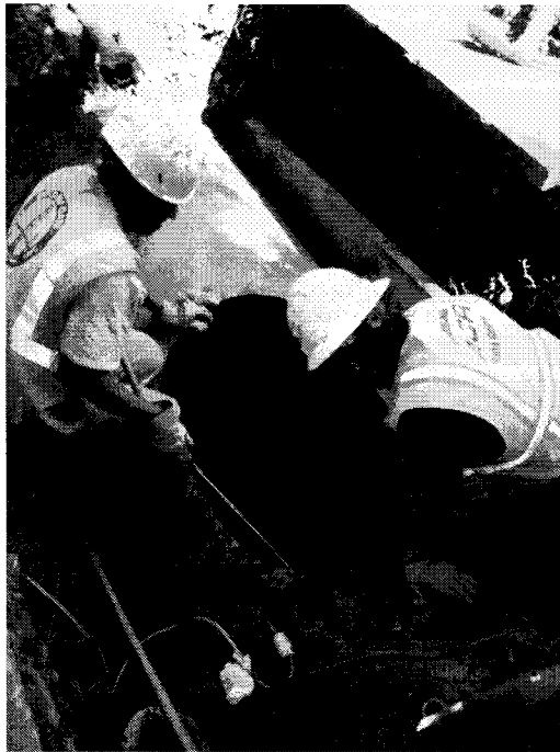
TANK READY TO BE REMOVED FROM EXCAVATION
