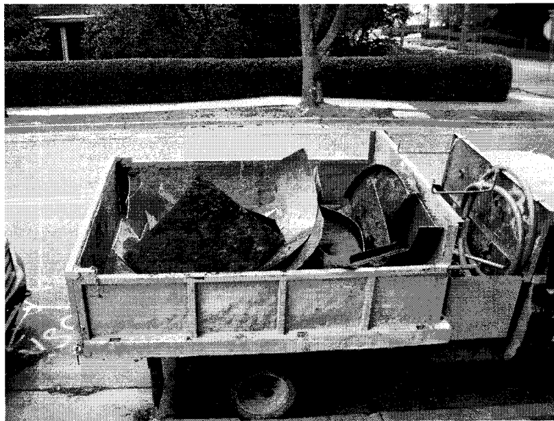
TANK CUT INTO PIECES READY TO BE TRANSPORTED FOR DISPOSAL
