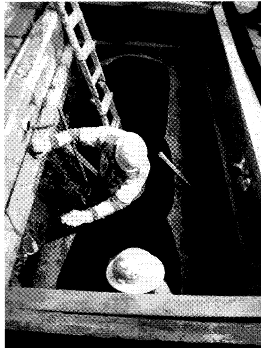
TANK READY TO BE REMOVED FROM EXCAVATION
