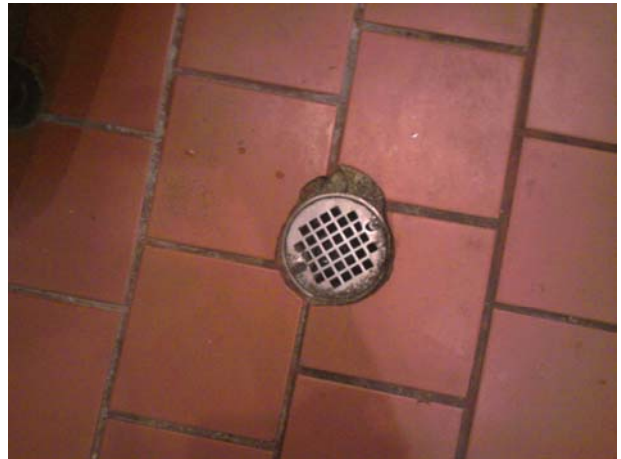
20. One of several floor drains located within 1540 Park Street.
