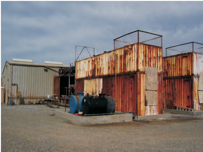
Photograph 1: Engine generator building, evaporators & AST's (View to the northwest).
