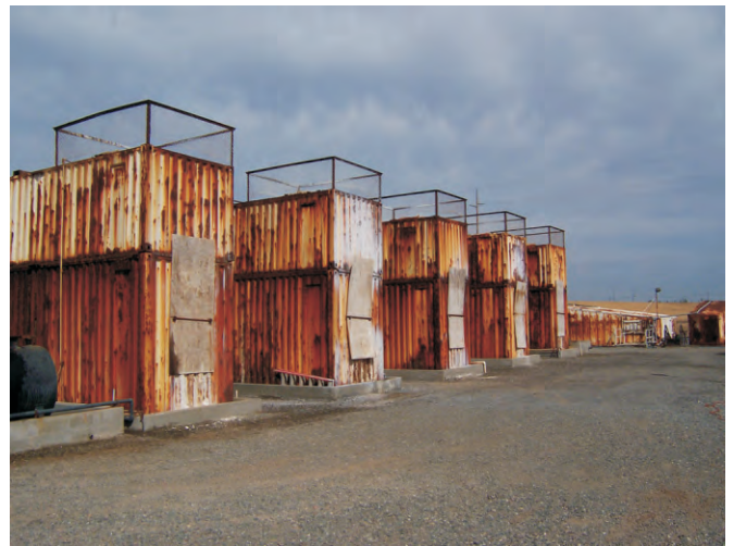
Photograph 10: Evaporators (View to the northwest).
