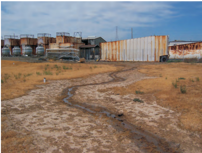
Photograph 11: Runoff from subject property onto adjacent property to the northeast (View to the southwest).
