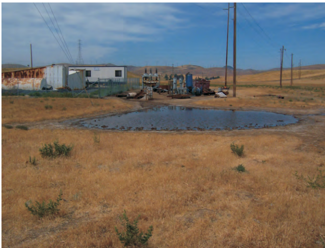
Photograph 9: Pool of liquid that overflowed from surface impoundment (View to the southwest).
