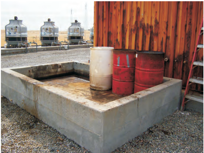
Photograph 5: 55-gal containers located within concrete secondary containment (View to the southeast).
