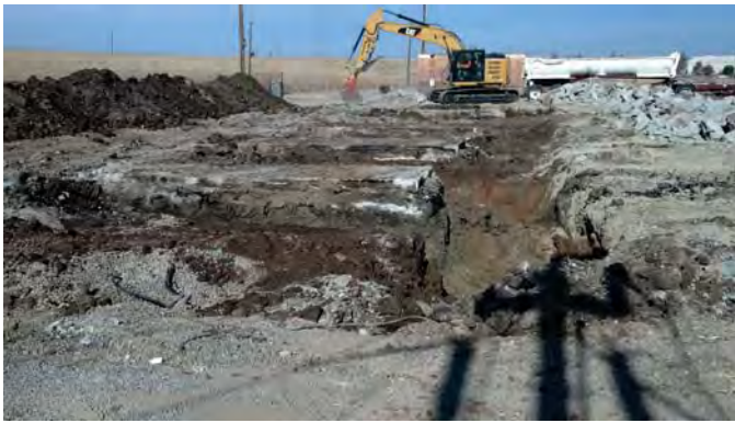
Photograph15: Demolition of Engine Isolation Pads (View to the northwest).
