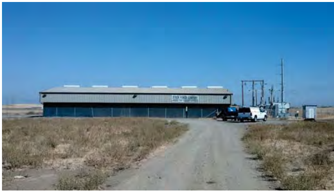
Photograph 1: Site Conditions Prior to Building Demolition & Remedial Excavation Activities (View to the northeast).
