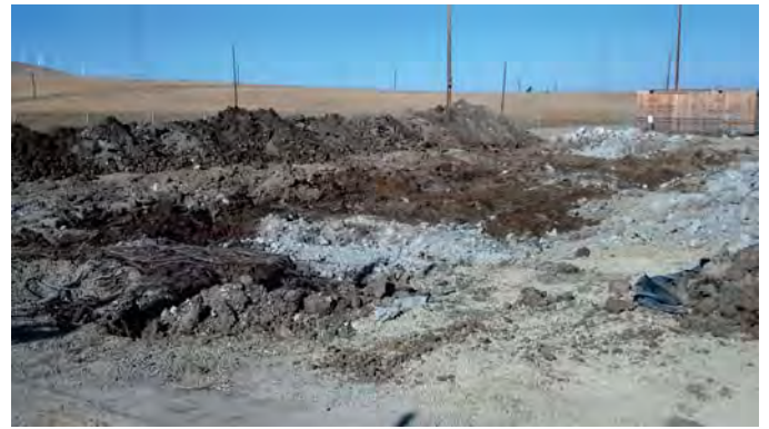
Photograph 16: Excavation After Removal of Engine Isolation Pads (View to the northwest).
