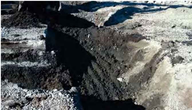
Photograph 11: Soil Excavation (View to the northwest).
