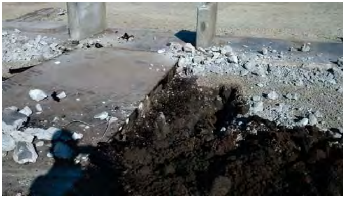
Photograph 9: Building Slab Demolition and Soil Excavation (View to the northeast).
