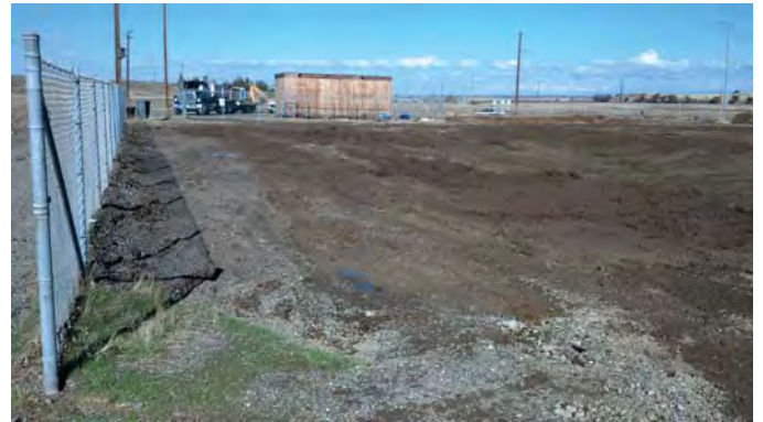
Photograph 18: Completion of Remedial Activities, Finished Grade (View to the north).
