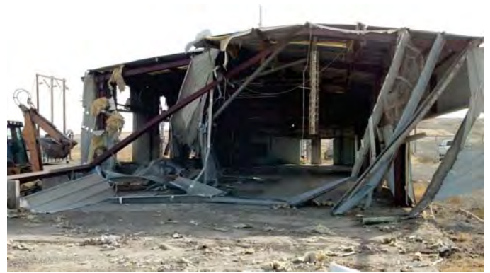
Photograph 4: Completion of Remedial Activities, Finished Grade (View to the southeast).
