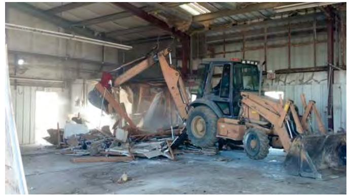
Photograph 2: Building Demolition (View to the south).
