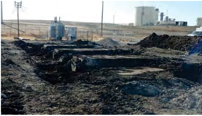
Photograph13: Demolition of Engine Isolation Pads (View to the south).
