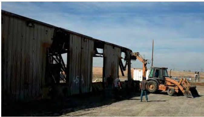
Photograph 3: Building Demolition (View to the northwest).
