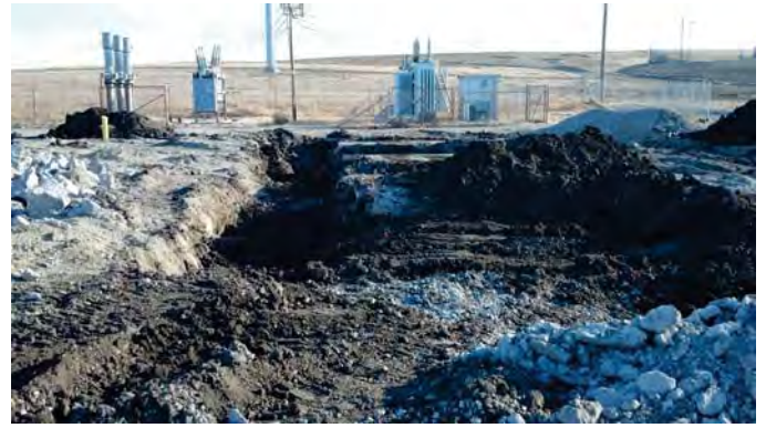
Photograph 14: Demolition of Engine Isolation Pads (View to the southeast).
