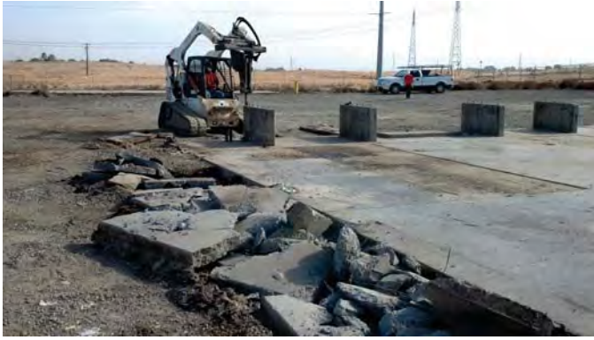
Photograph 7: Building Slab Demolition (View to the southeast).
