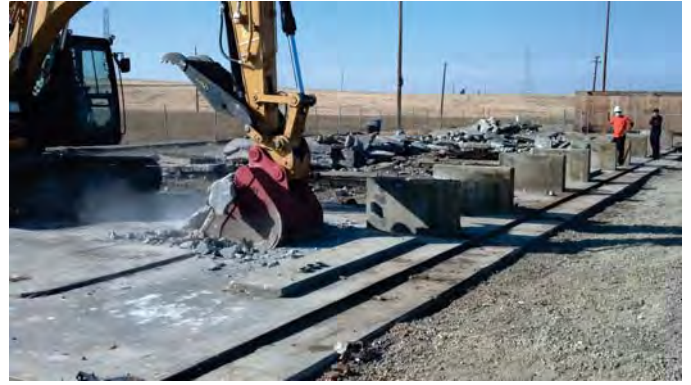
Photograph 8: Building Slab Demolition (View to the northwest).
