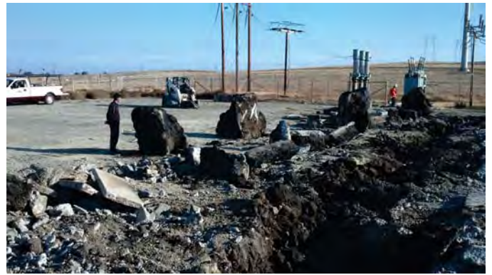
Photograph 10: Building Slab Demolition, Removal of Foundation Piers (View to the southeast).
