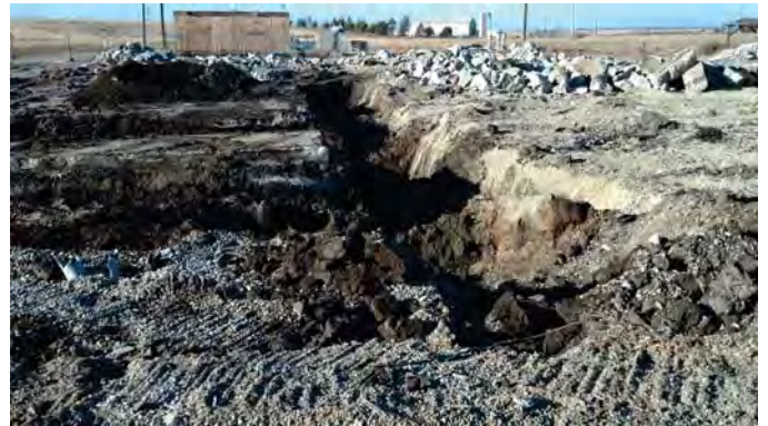
Photograph 12: Building Slab Demolition and Soil Excavation (View to the northwest).
