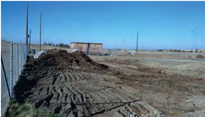
Photograph 17: Soil Stockpile (View to the north).
