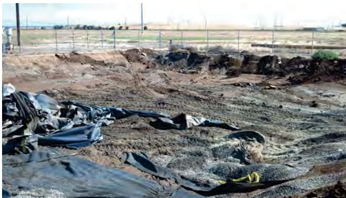
Photograph 5: Exposed Native Soil Beneath Secondary Liner (View to the northeast).
