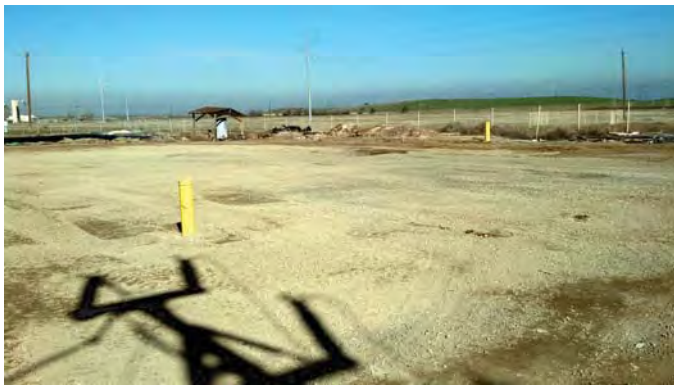
Photograph 3: Completion of Remedial Activities, Finished Grade (View to the northeast).
