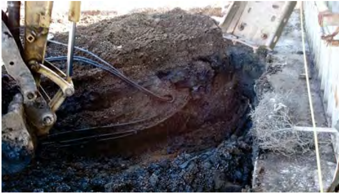
Photograph 11: Electrical Conduits at Southeast Corner of Building (View to the south).
