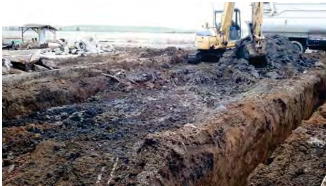
Photograph 25: Excavation of East-end of Evaporator Pad #2 (View to the northeast).
