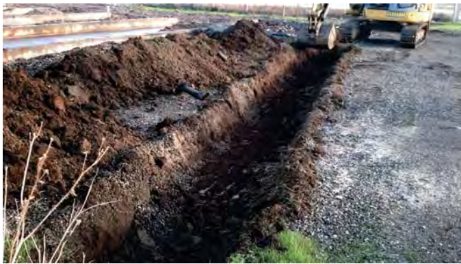
Photograph 5: Initial Excavation Along South Excavation Boundary (View to the east).
