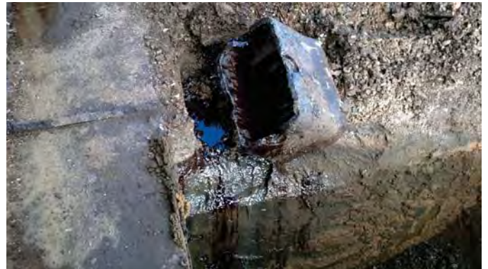
Photograph 16: Building Ground Rod Box Between Evaporator Pads #2 & 3 Containing Free-Phase Product (View to the north).
