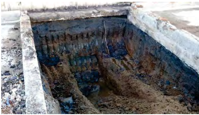
Photograph 17: Excavation Between Evaporator Pads #2 & 3 (View to the west).
