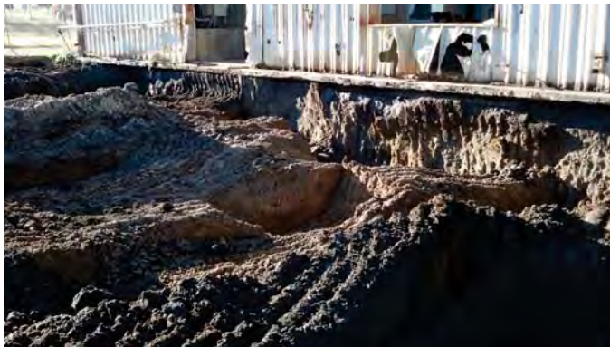
Photograph 27: Remedial Excavation Near Evaporator Pad #2 (View to the southwest).
