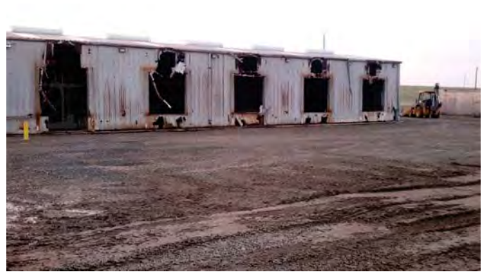
Photograph 4: Completion of Remedial Activities, Finished Grade (View to the northwest).
