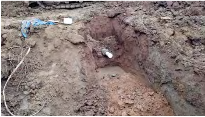
Photograph 29: Capped Secondary-Contained Conduit, Which Appears Connected to the Adjacent Surface Impoundment (View to the northeast).
