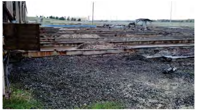
Photograph 2: Site Conditions Prior to Remedial Excavation Activities (View to the north).
