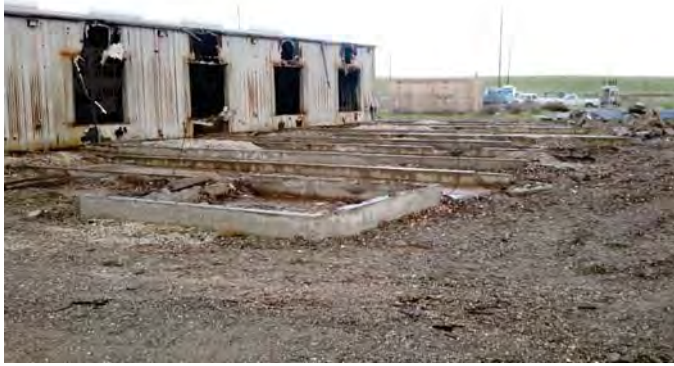
Photograph 1: Site Conditions Prior to Remedial Excavation Activities (View to the northwest).
