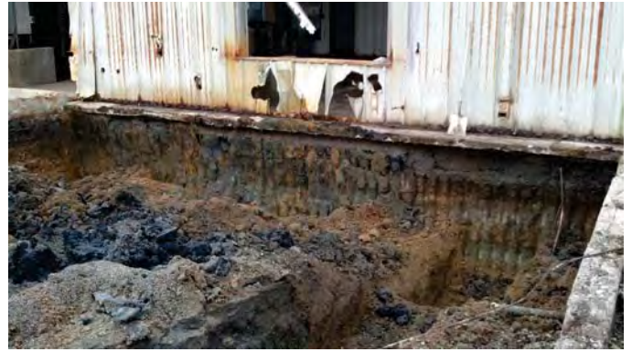
Photograph 24: Excavation of West-end of Evaporator Pad #2 (View to the southwest).
