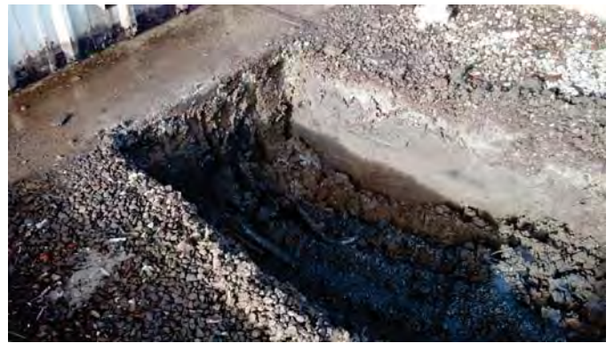
Photograph 6: Excavation Between Evaporator Pads #2 & #3 (View to the northwest).
