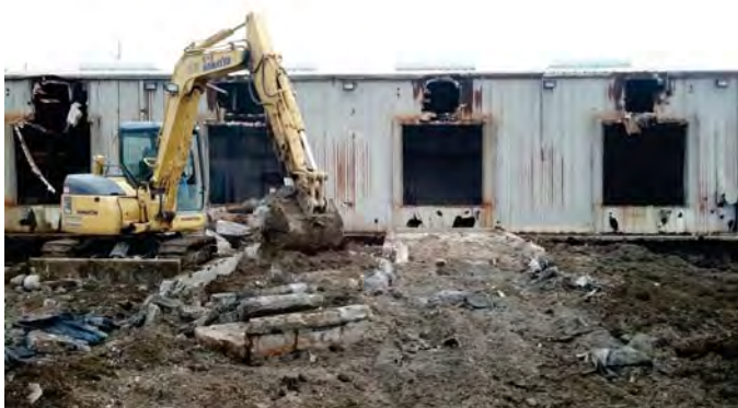
Photograph 21: Removal of Evaporator Pad #3 (View to the west).
