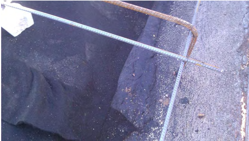
Photograph 1: Close-up view showing Liquid Boot® barrier.
