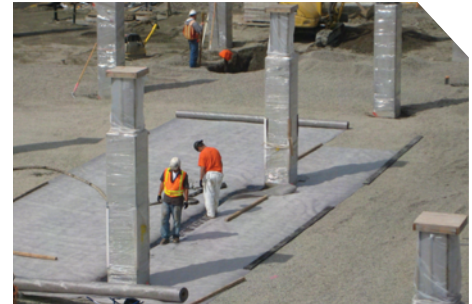
BaseFabric™ T-60 is a needle-punched, non-woven geotextile with superior tensile strength and puncture resistance.
