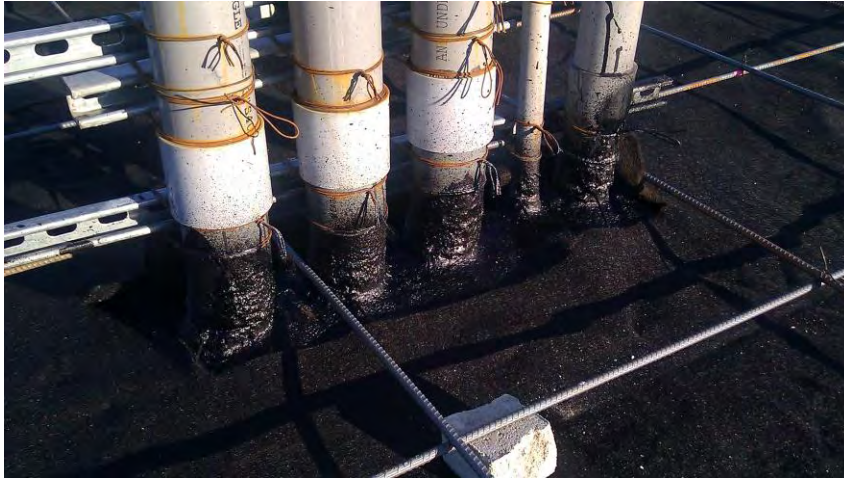
Photograph 2: View showing Liquid Boot® seal around utility piping.
