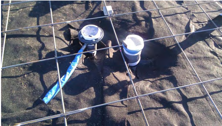
Photograph 3: View showing riser fitting above geo-textile fabric.
