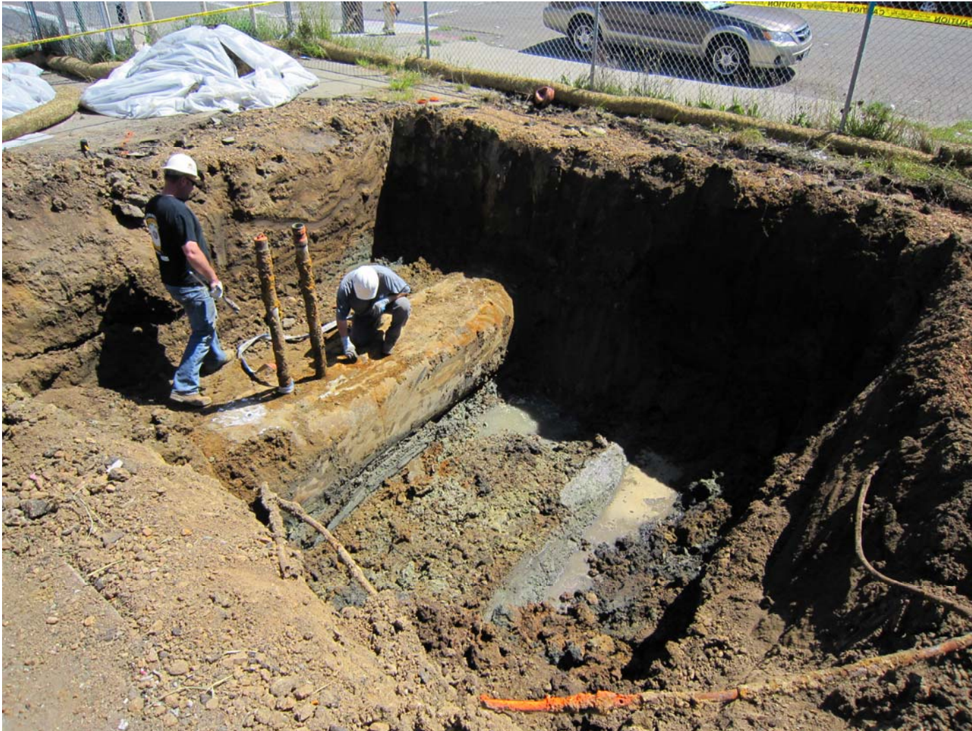
Excavation and Removal of UST#1 and UST#2
