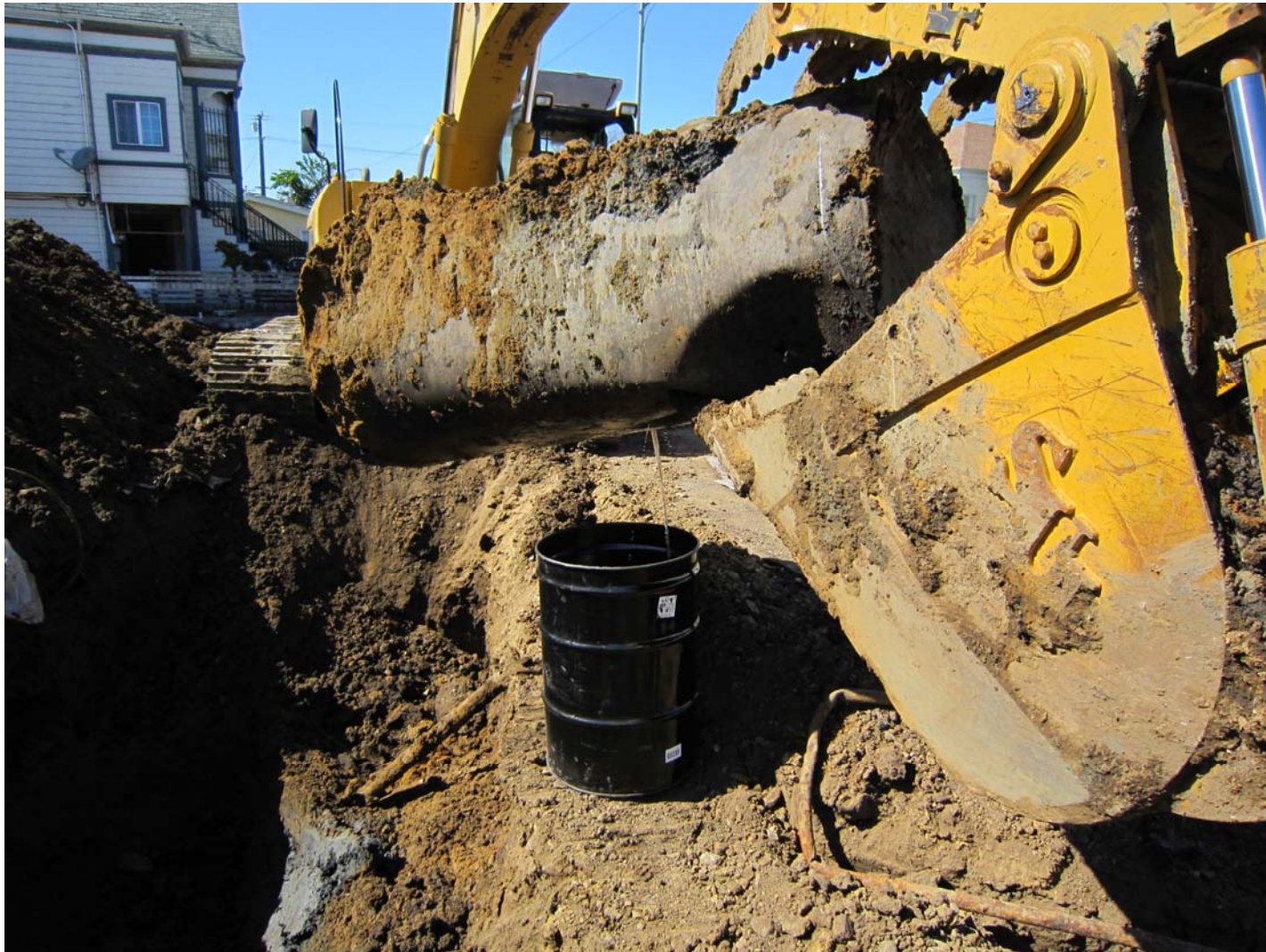
Removal of UST#3 and Drainage of Leftover Rinsate Water
