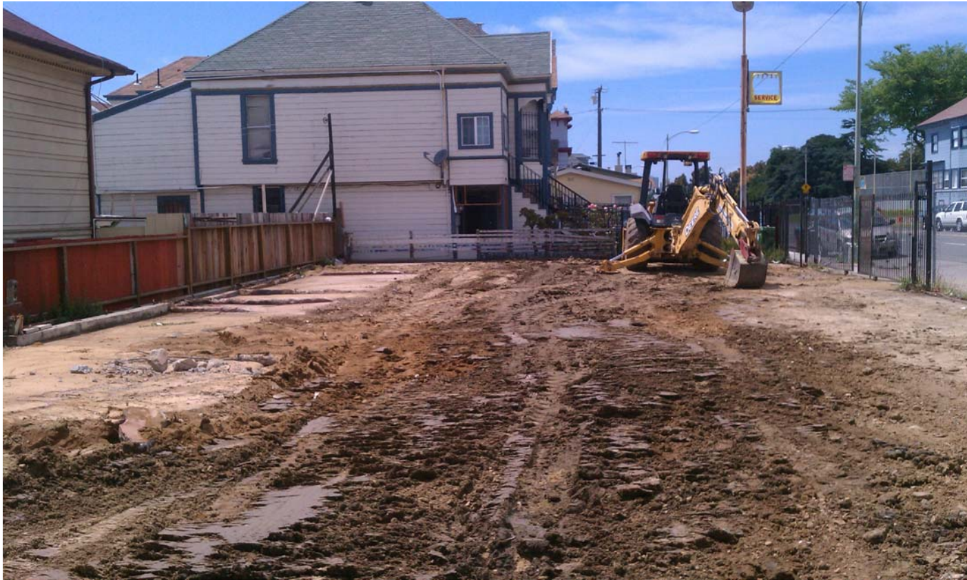
Site Surface Following Removal of Soil Stockpiles
