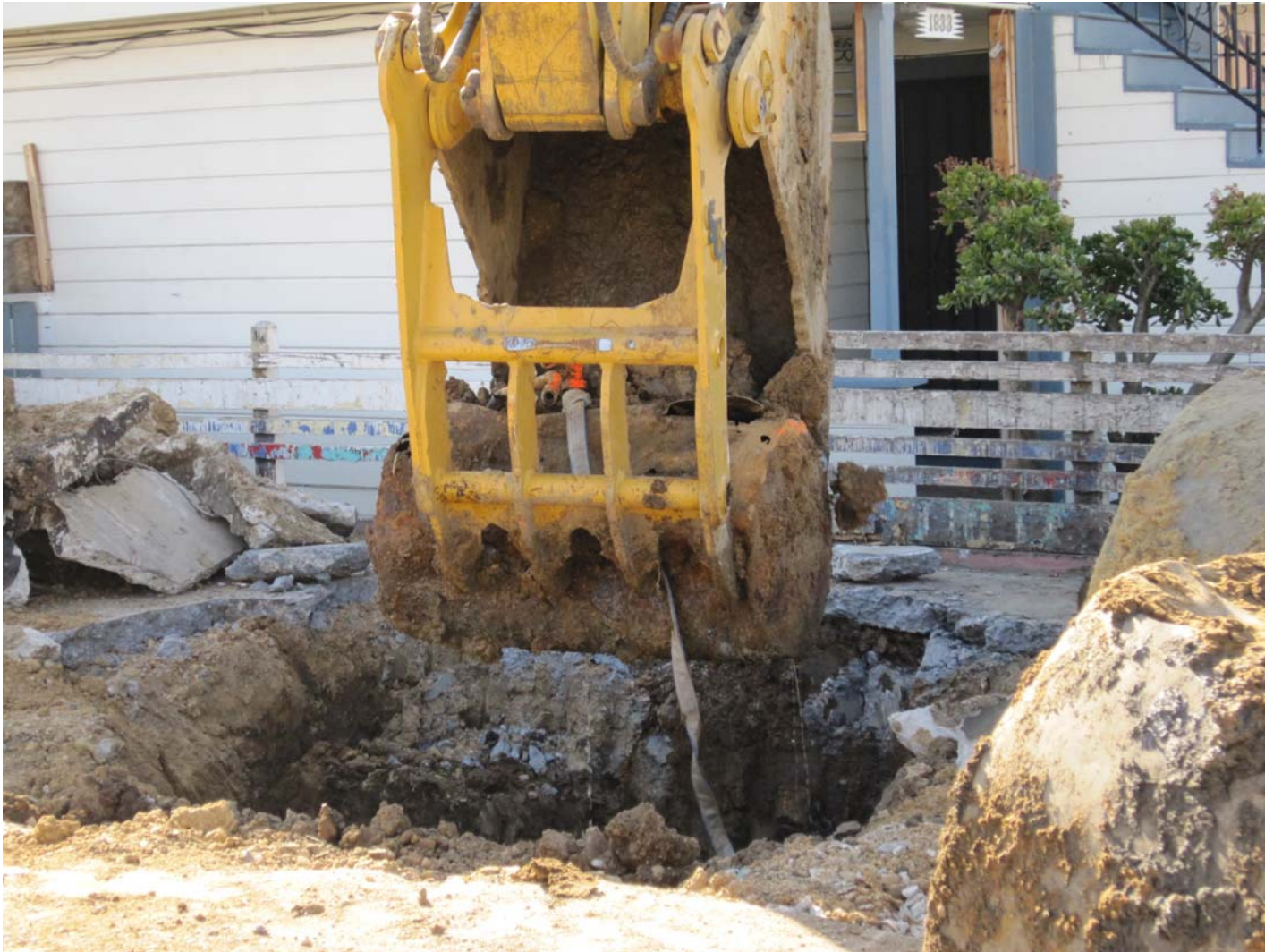
Removal of UST#4
