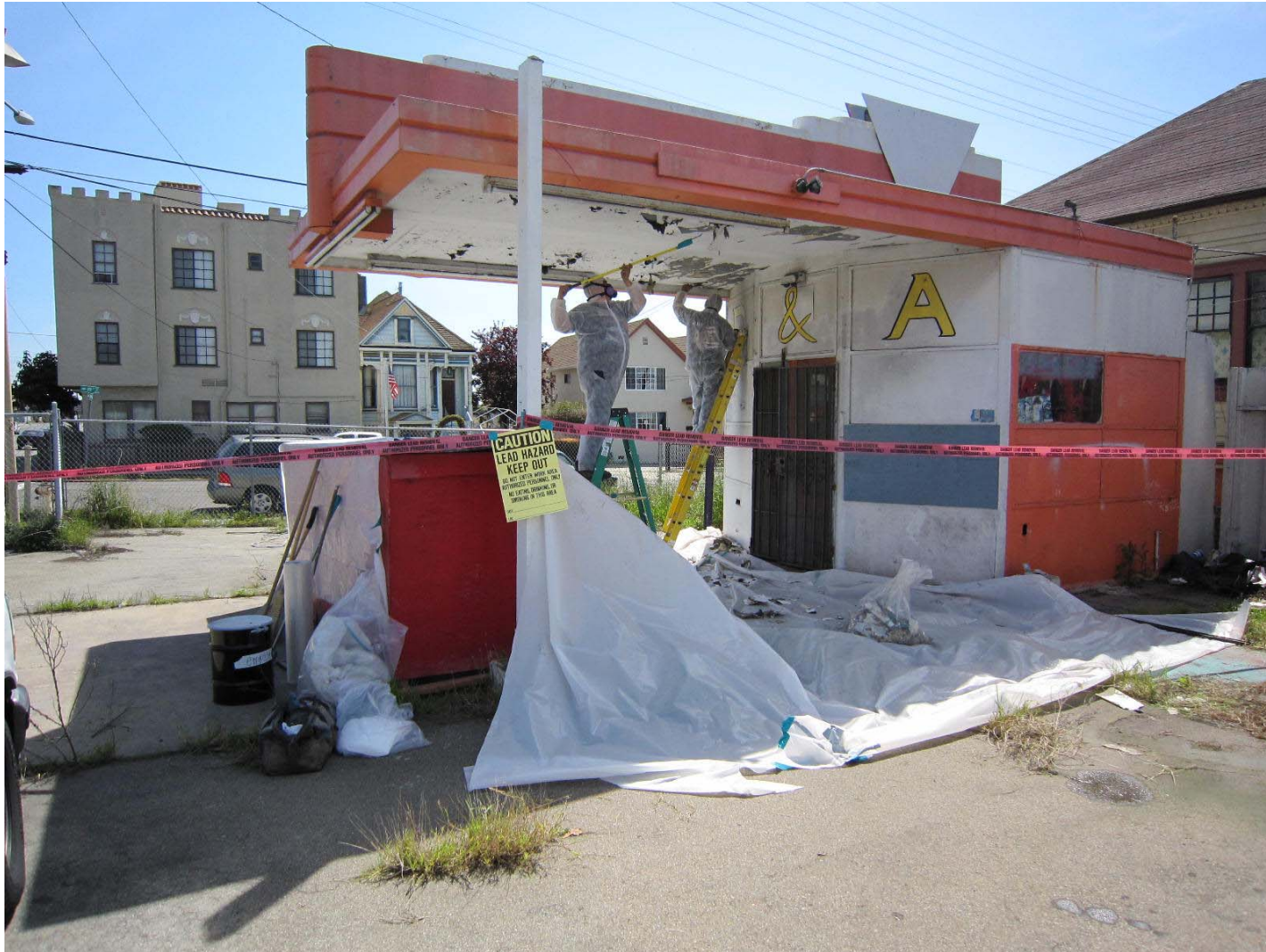
Abatement of Lead Based Paint Prior to Building Demolition
