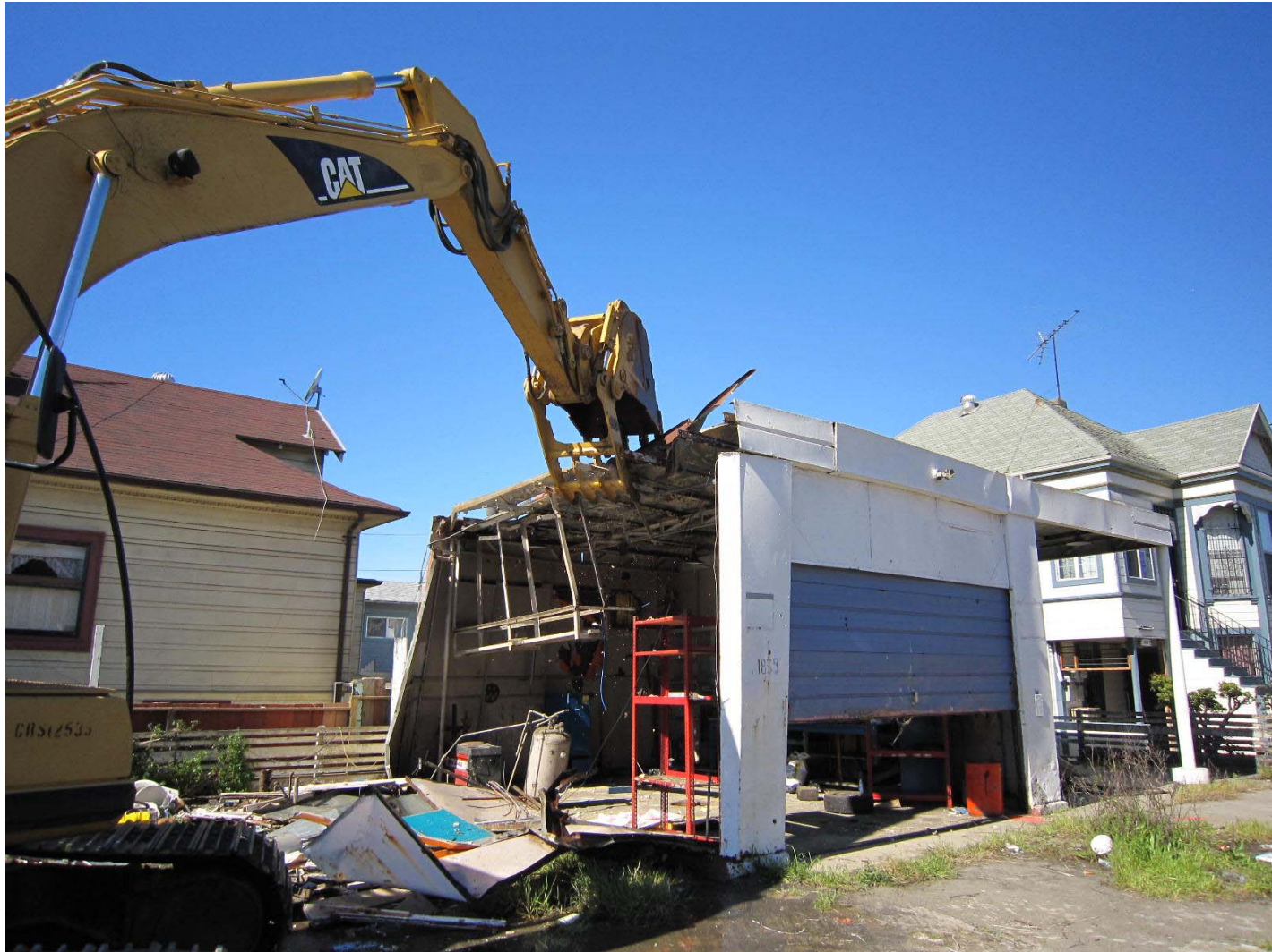
Demolition of Former Auto Service Garage and Canopy
