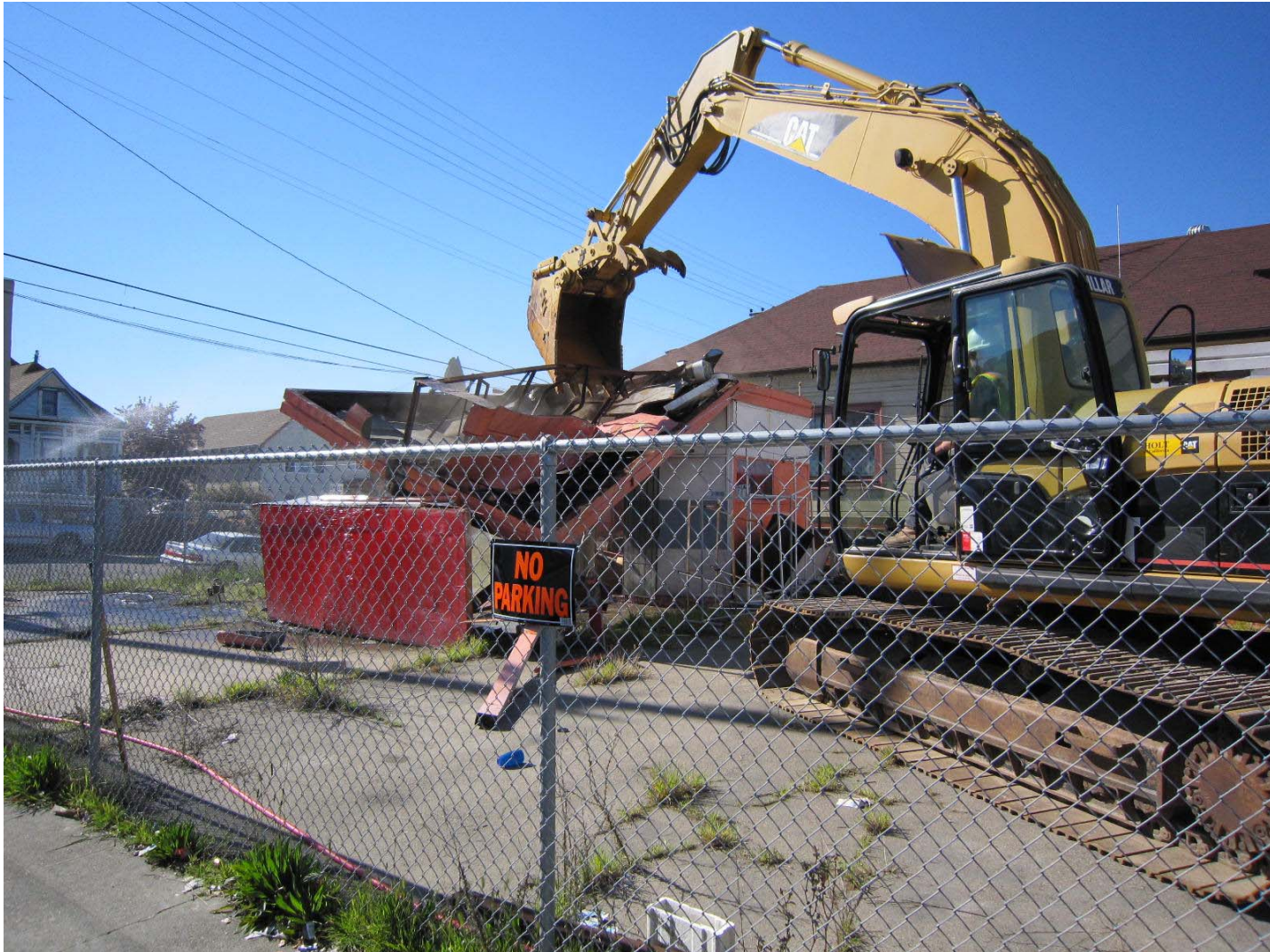
Demolition of Former Retail Building and Canopy
