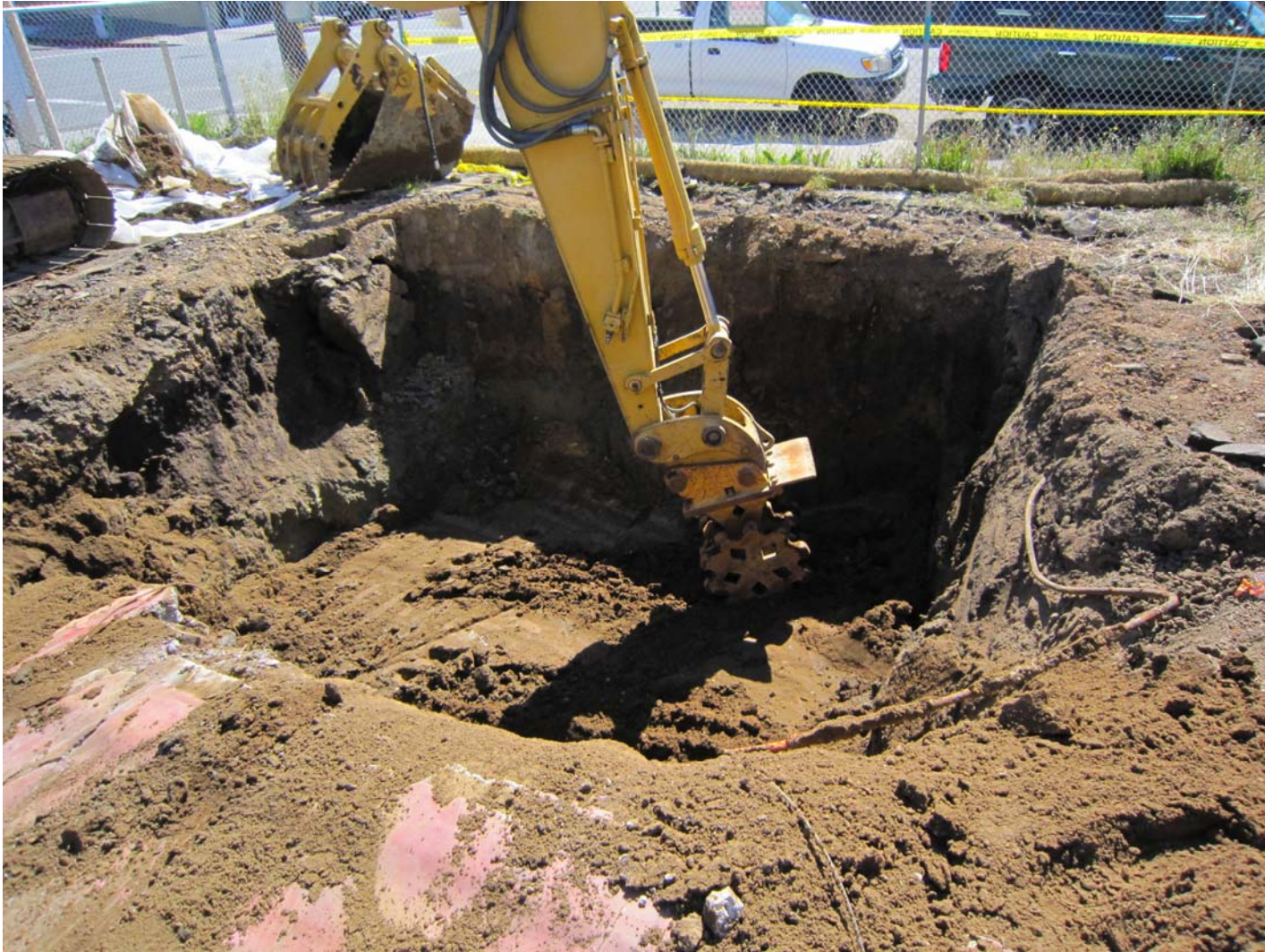
Backfill and Compaction of Excavations
