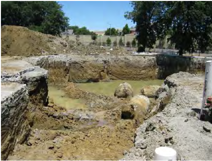
VIEW OF EXCAVATIONS #1 AND #3 LOOKING NORTH
