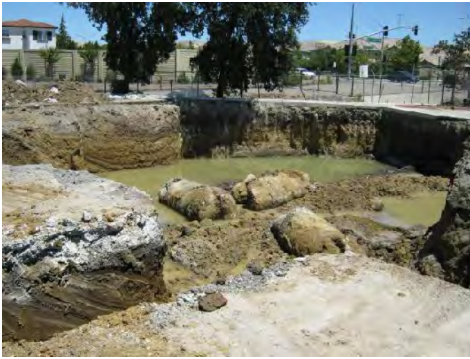
VIEW OF EXCAVATION #3 LOOKING NORTHEAST
