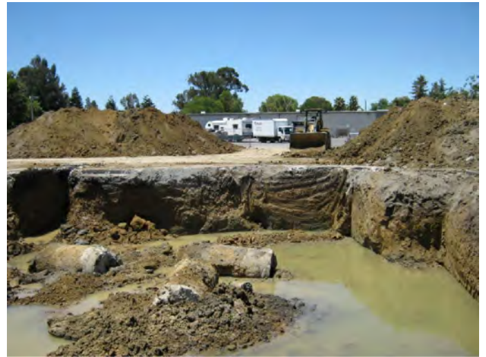
VIEW OF EXCAVATIONS #1 AND #3 LOOKING NORTH
