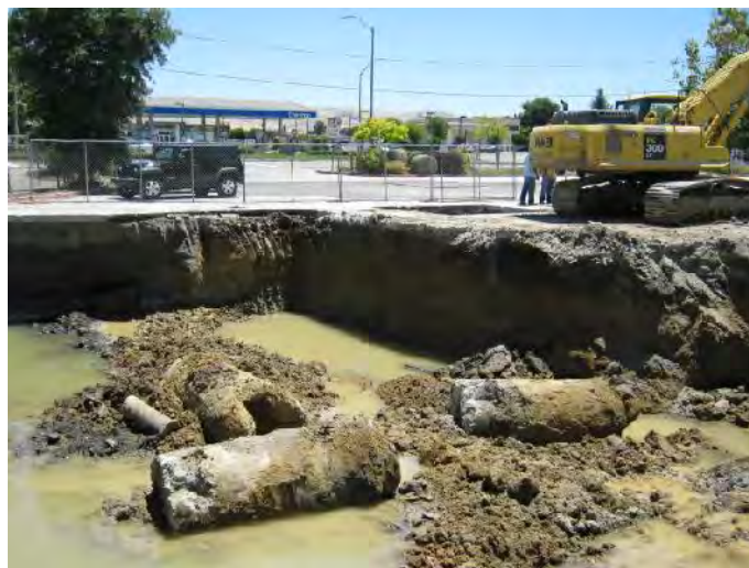
VIEW OF EXCAVATIONS #1 AND #4 LOOKING SOUTHEAST
