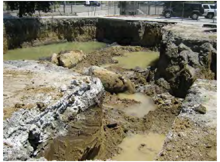
VIEW OF EXCAVATIONS #1 AND #3 LOOKING EAST
