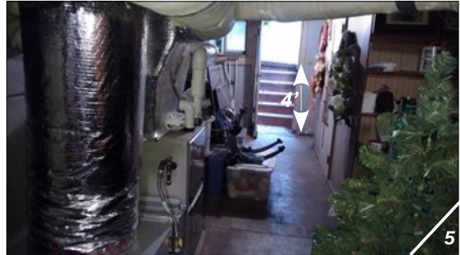
Photograph No. 6 – West view of interior of basement showing location of existing product/return piping (capped @ 4" above floor surface) associated with former UST oil burner system (WGE, 8/9/17).
