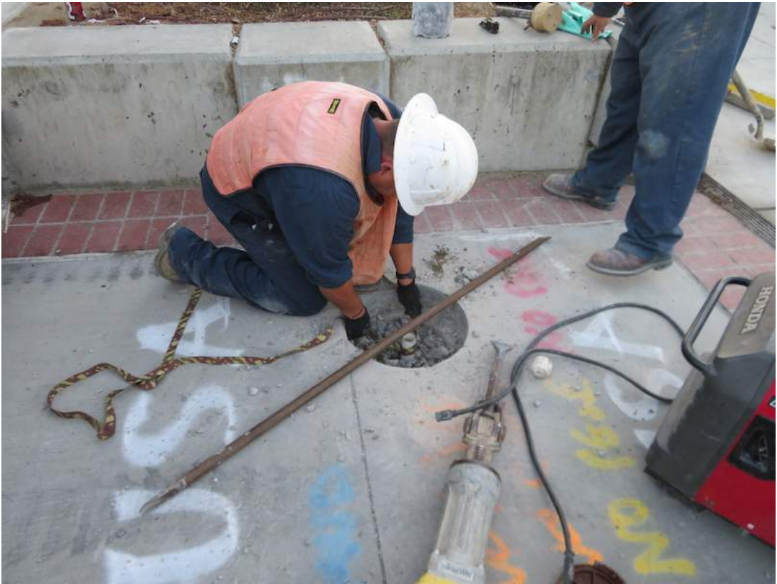
Photograph 3 – Clearing concrete from around well head.
