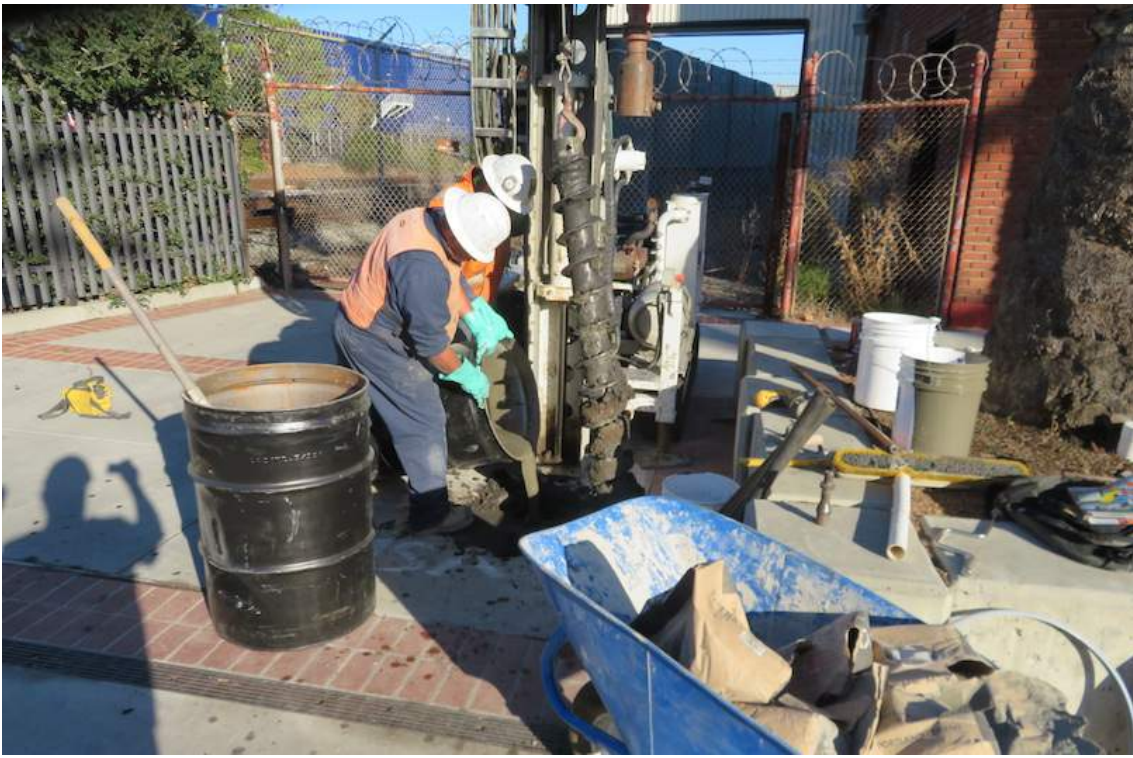
Photograph 7 – Filling in hole with grout.
