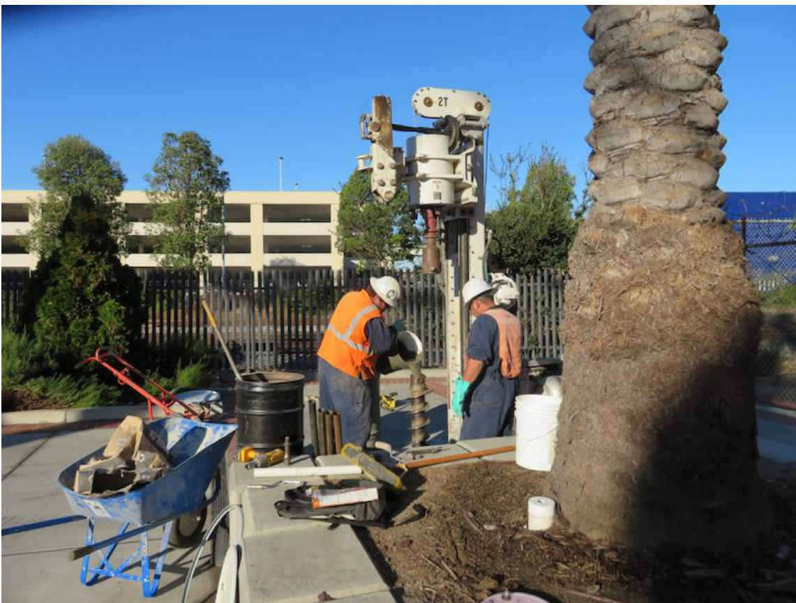
Photograph 6 - Pouring grout into auger to reach the bottom of the hole.
