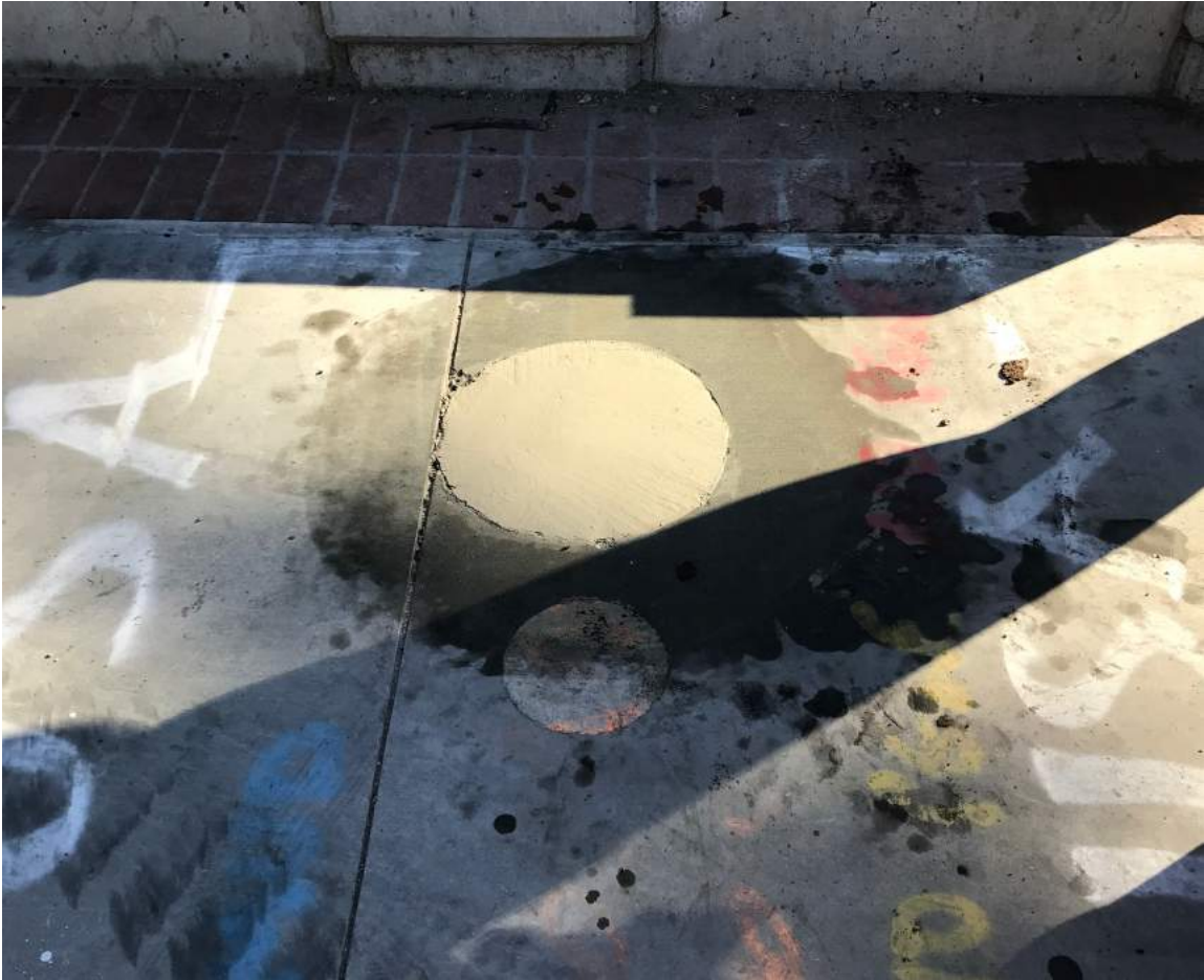
Photograph 8 – Completed concrete surface over former monitoring well location.
