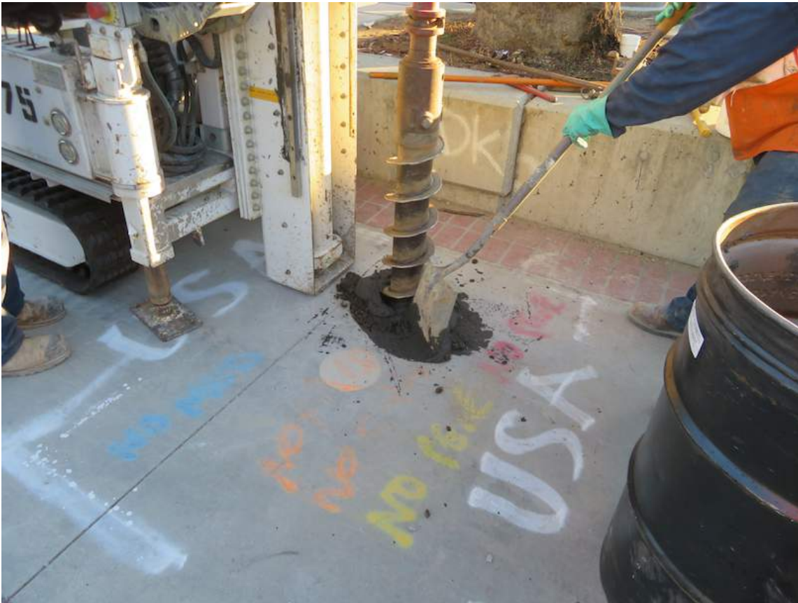
Photograph 5 – Close-up of drilling out well material.
