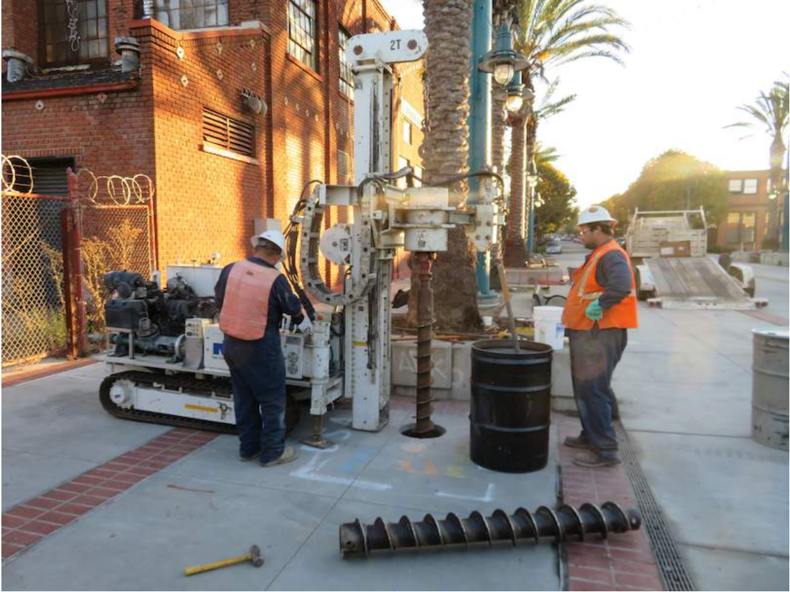
Photograph 4 – Using 8-inch diameter auger to drill out well material.
