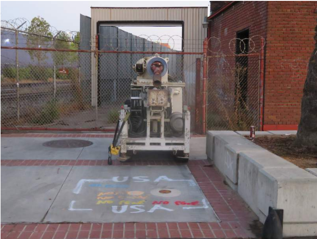
Photograph 1 – Limited access rig in position to begin well abandonment.
