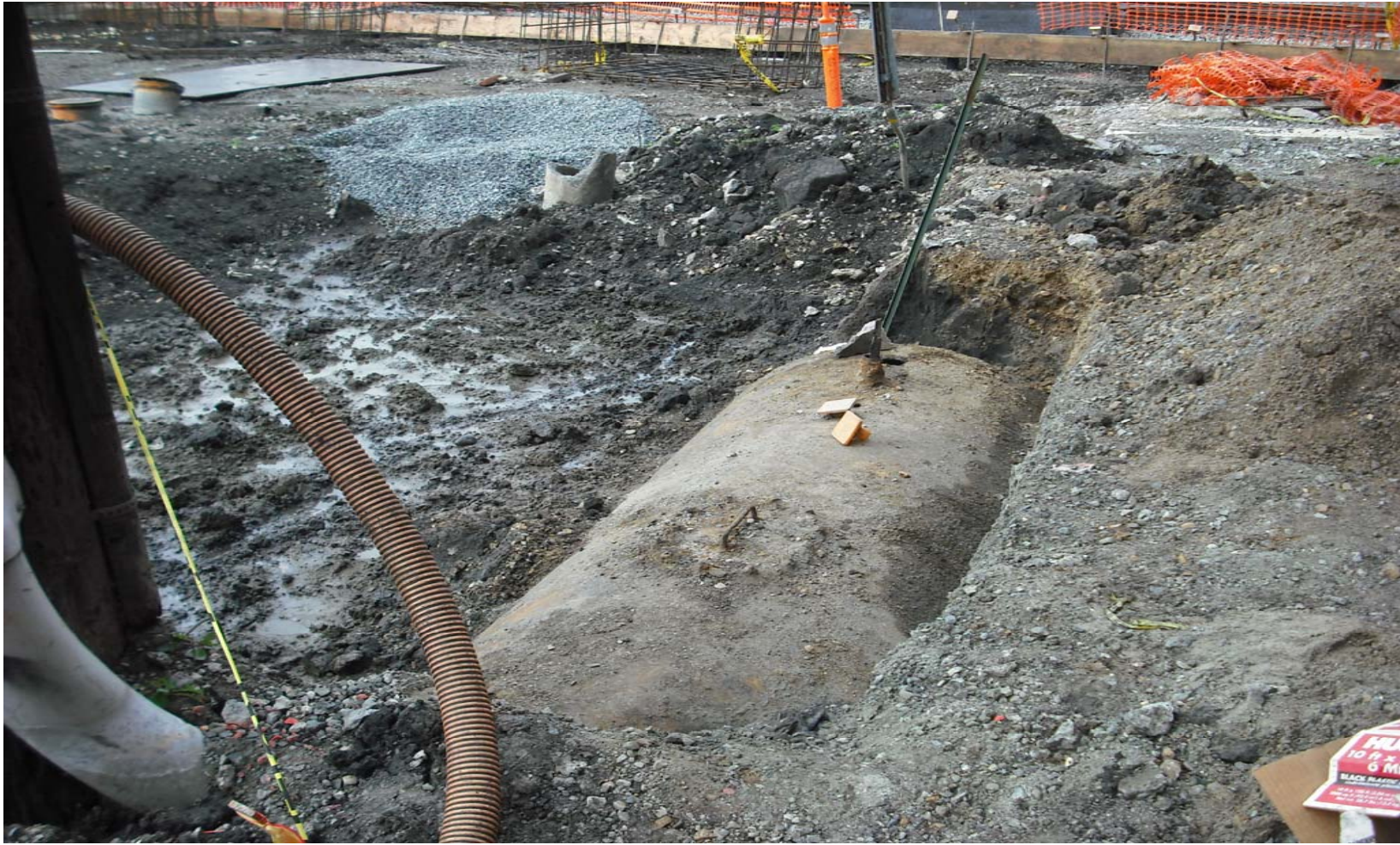
Construction excavation located to the south of UST
