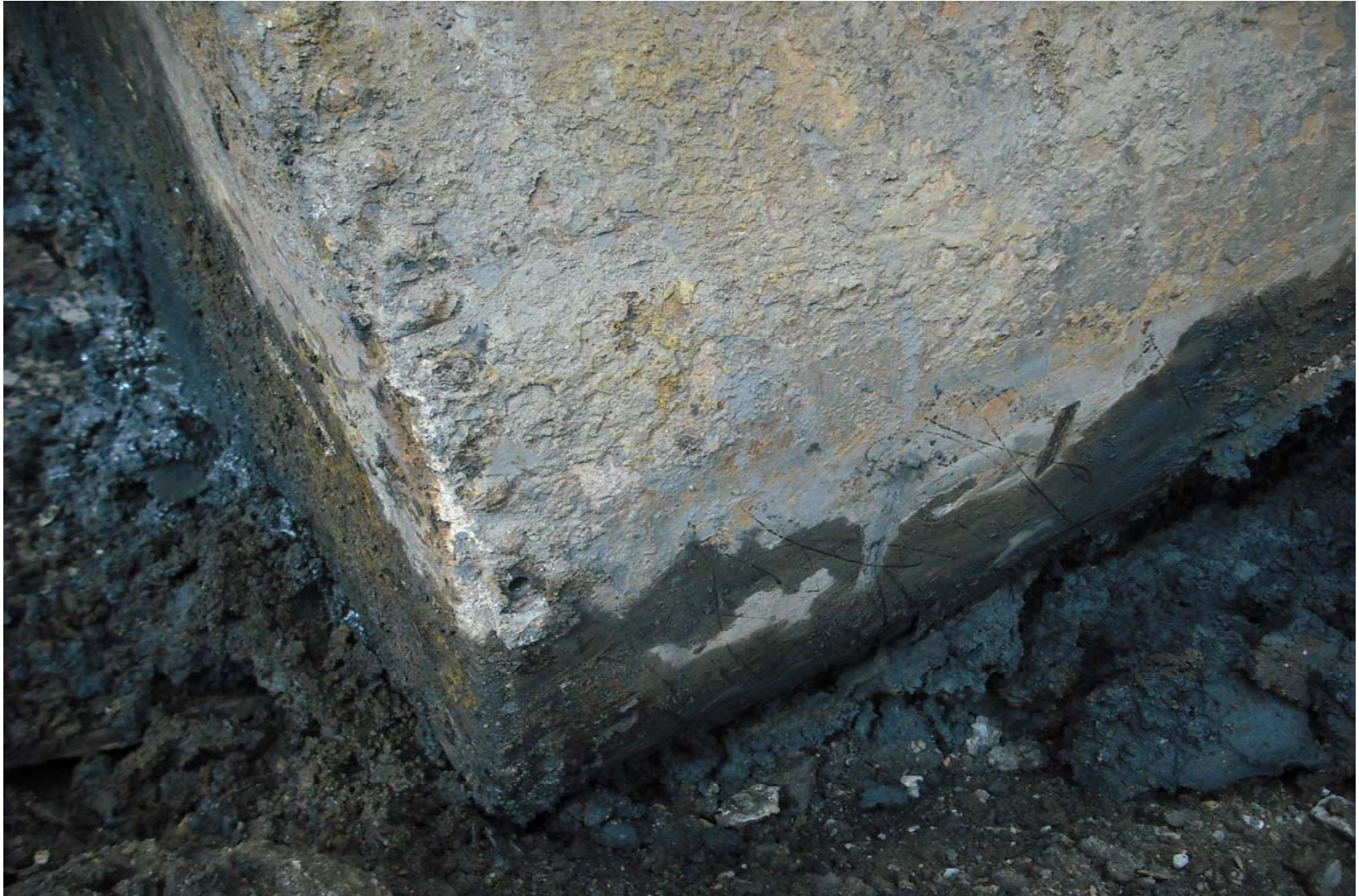
Missing rivet from UST
