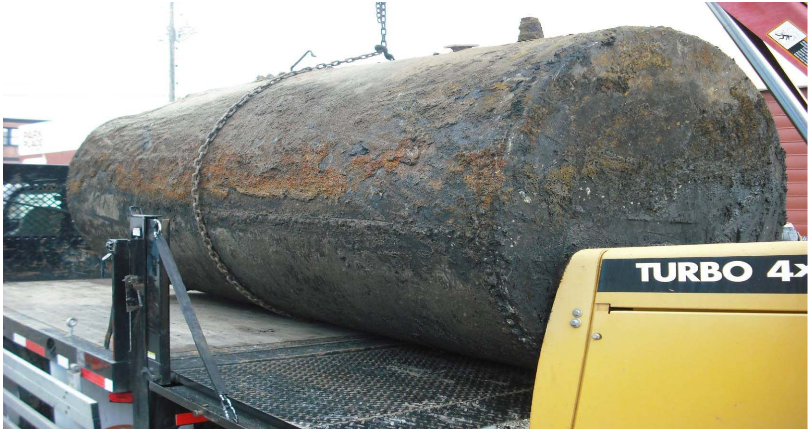
UST following removal
