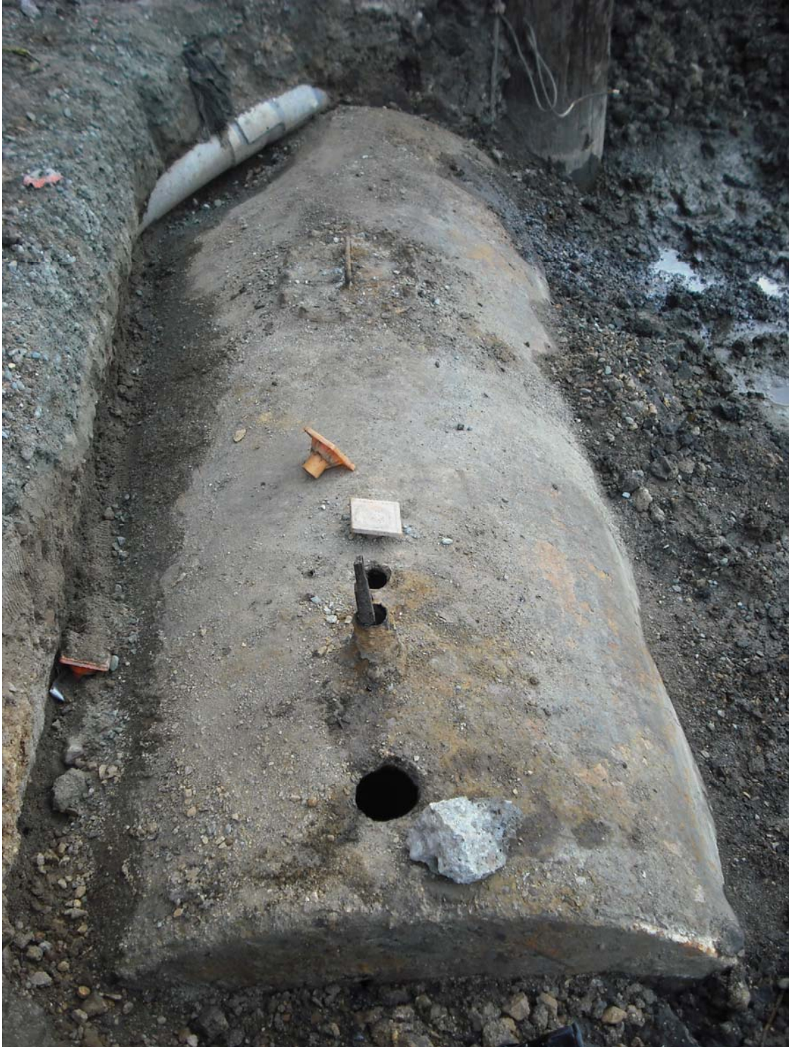
UST prior to removal
