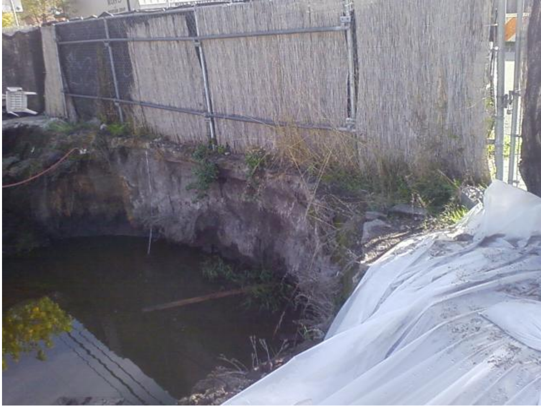
Plate 3. View of excavation sidewall where sample EX-3-S-W was collected
