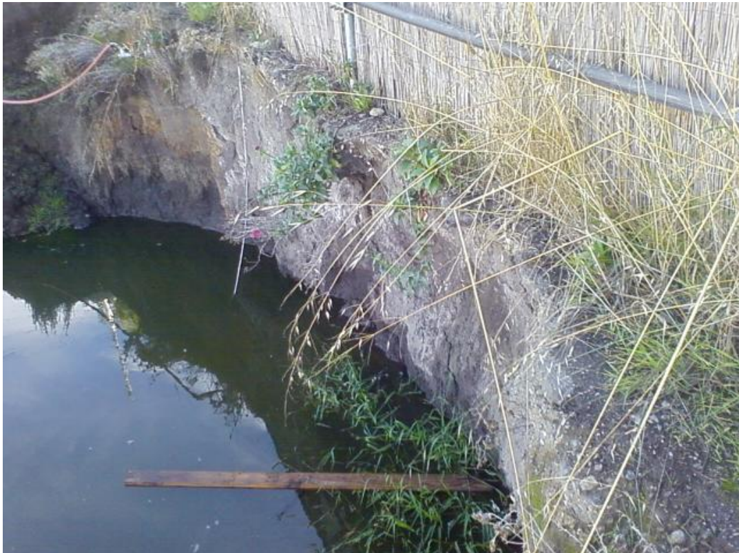
Plate 2. View of excavation sidewall where sample EX-3-S-W was collected
