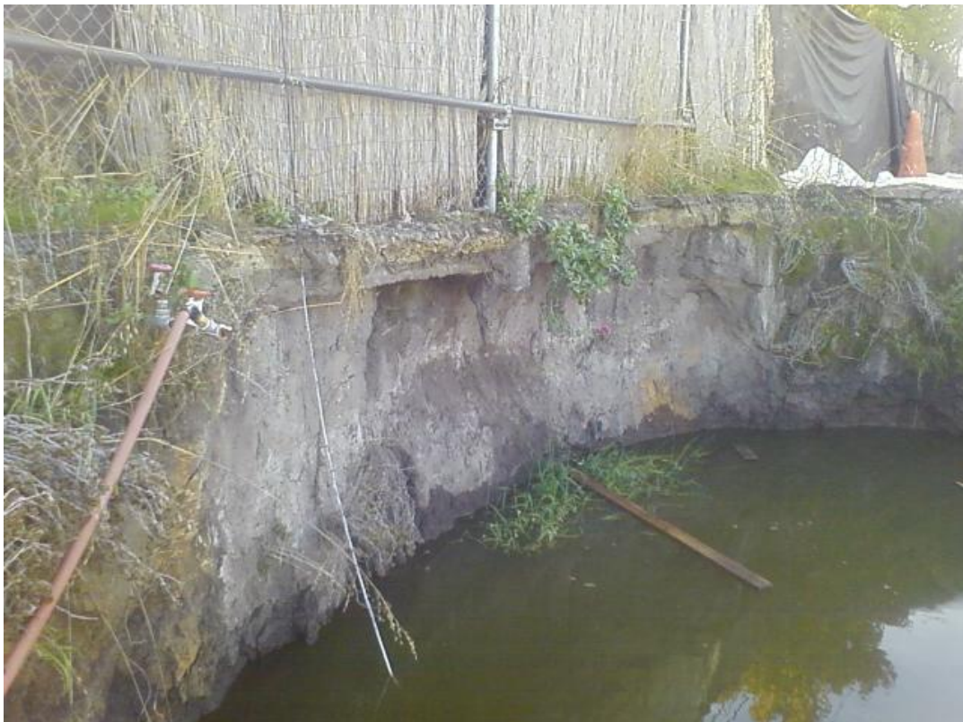
Plate 4. View of excavation sidewall where sample EX-3-S-W was collected
