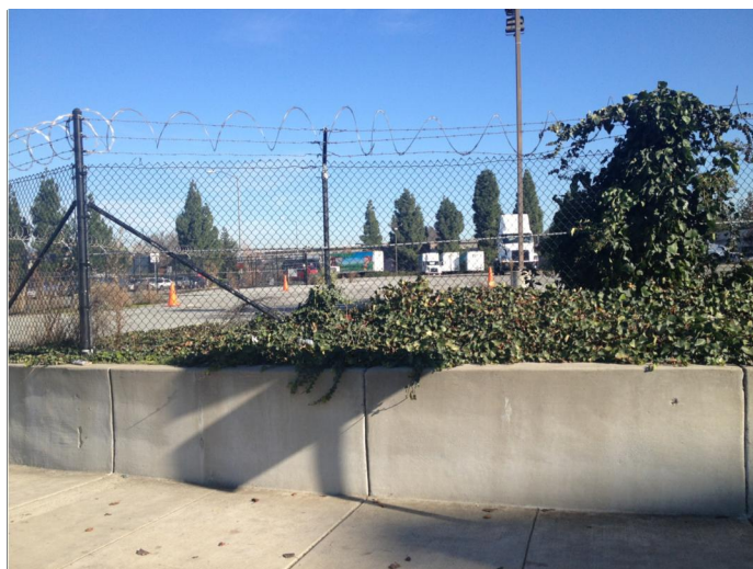
VIEW OF SITE AND VEGETATION BEHIND RETAINING WALL TAKEN FROM THE NORTHWEST CORNER FACING SOUTHEAST
