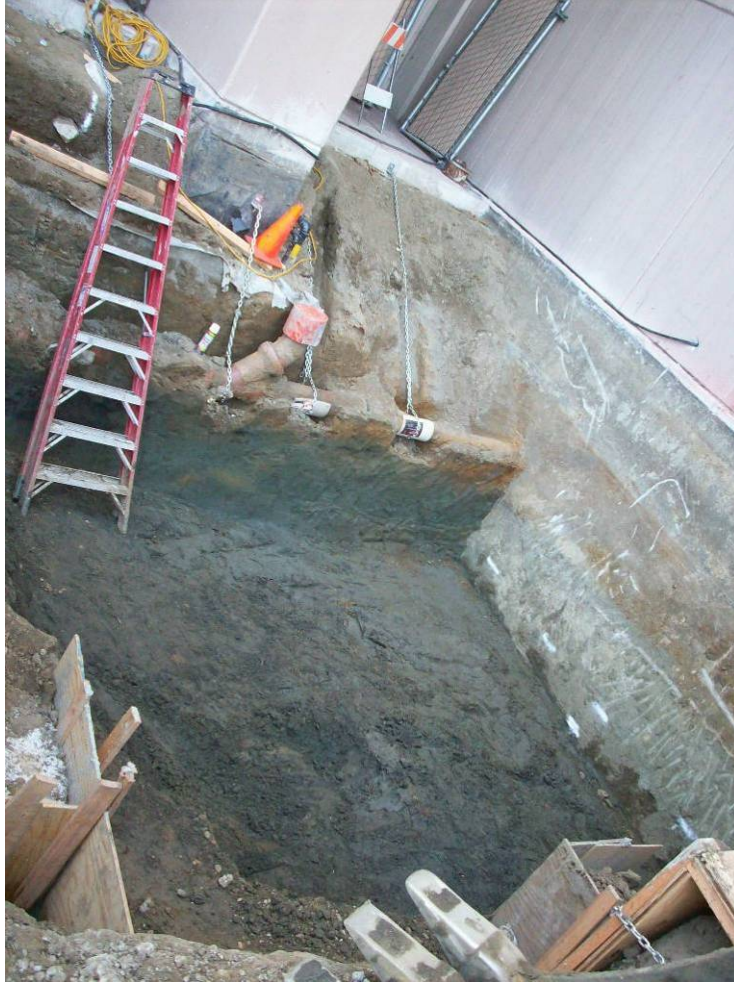
Photograph 2. The completed excavation to approximately 10 feet bgs.
