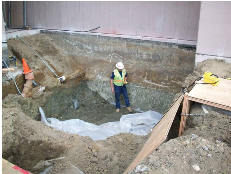
Photograph 1. Air monitoring inside the excavation at 9 feet bgs.
