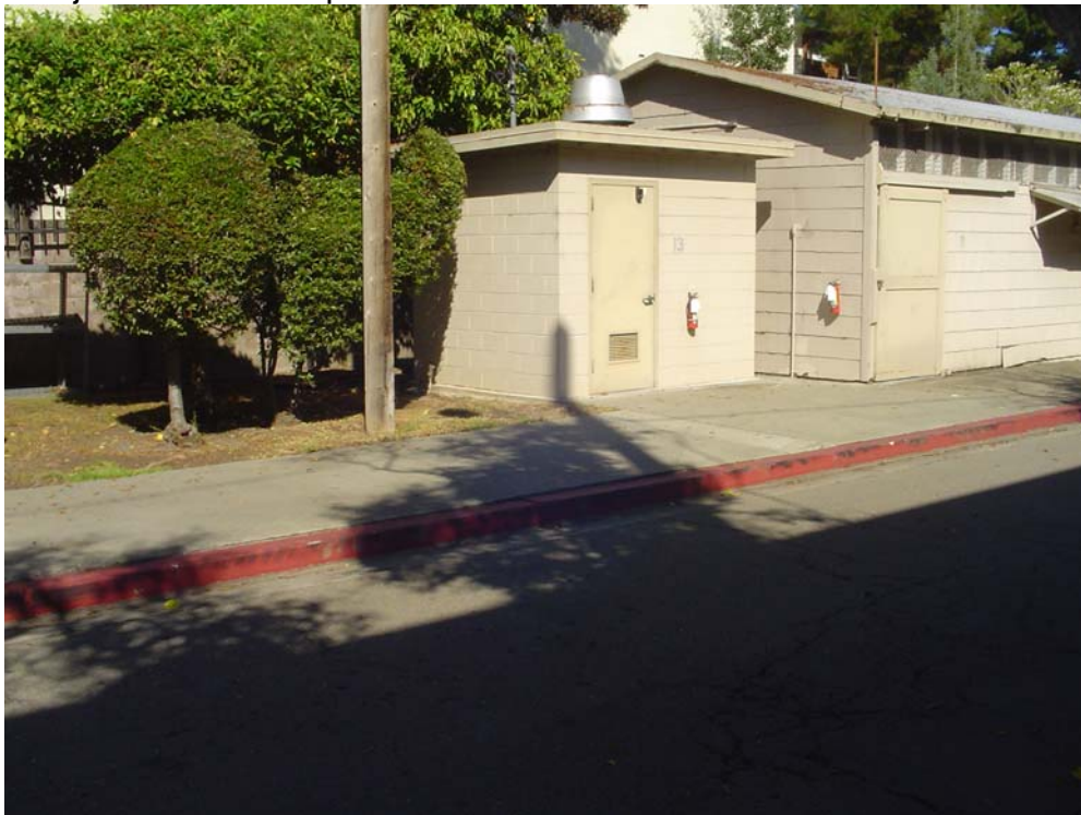
Elevator control room showing trench location on sidewalk. Excavation will extend from elevator building, across the street, to the control room.
