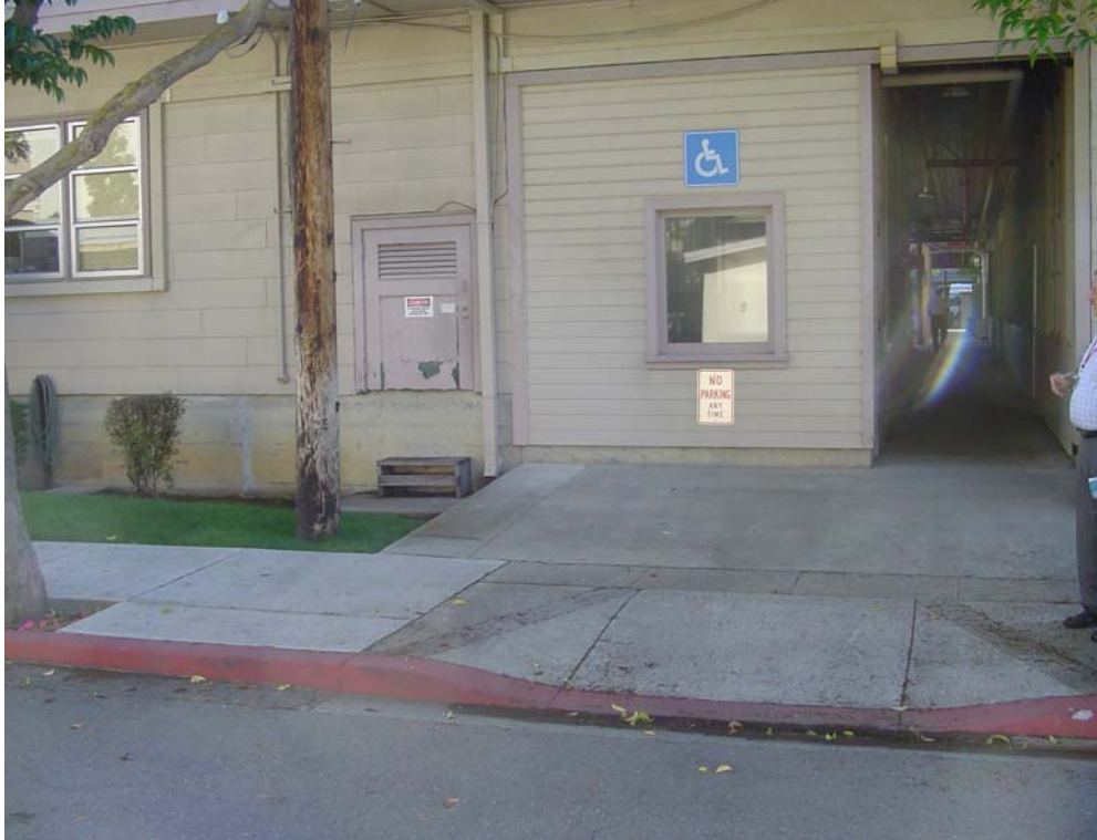
Elevator located on the other side of the window. Trench for hydraulic pipeline located adjacent to down spout.
