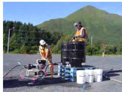
RegenOx Soil Mixing Application
