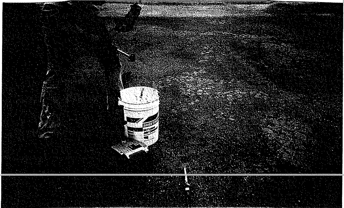
Above - Using two inch flight auger with pneumatic rotary hammer. Below - Using bucket auger to clean out hole.
