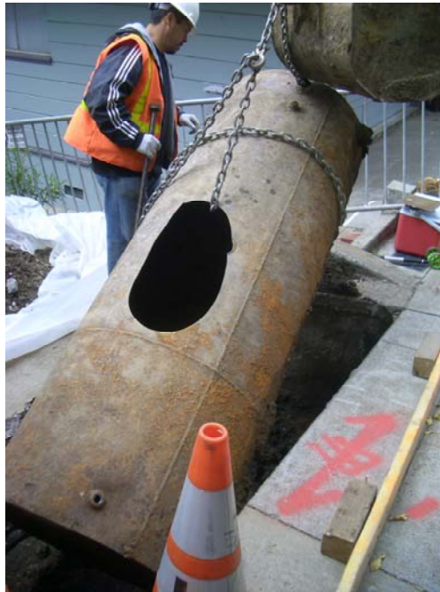
TANK READY TO BE REMOVED FROM EXCAVATION
