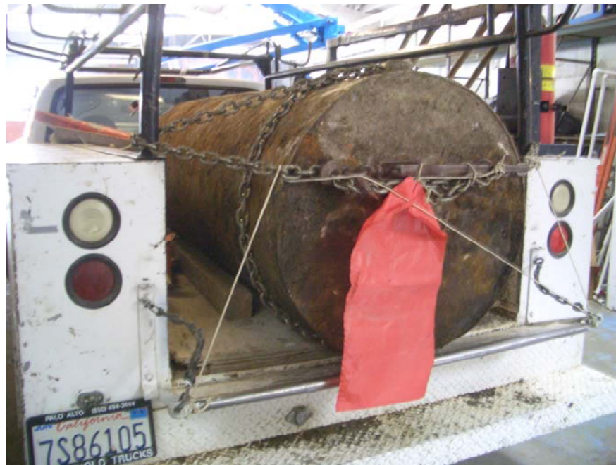
TANK READY TO BE TRANSPORTED FOR DISPOSAL
