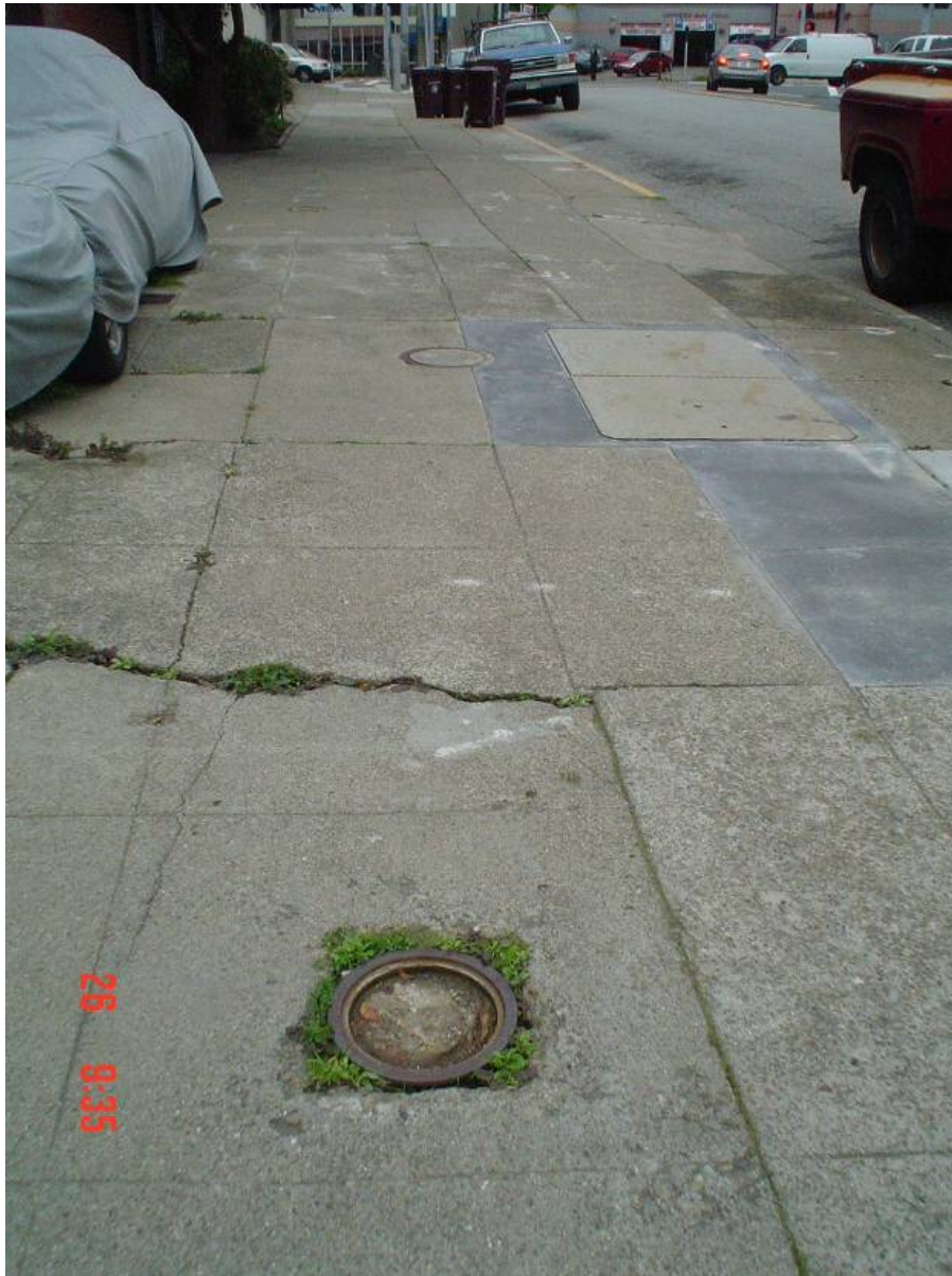
Plate 3: View east, along the sidewalk adjacent to the site, two decommissioned well boxes visible (possible locations of B-12 and B-11)
