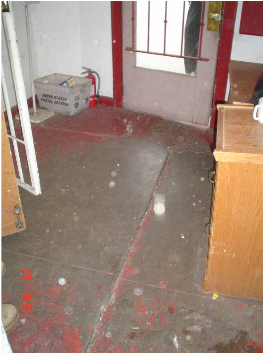
Plate 5: Proposed location for LDP-1 inside the site building
