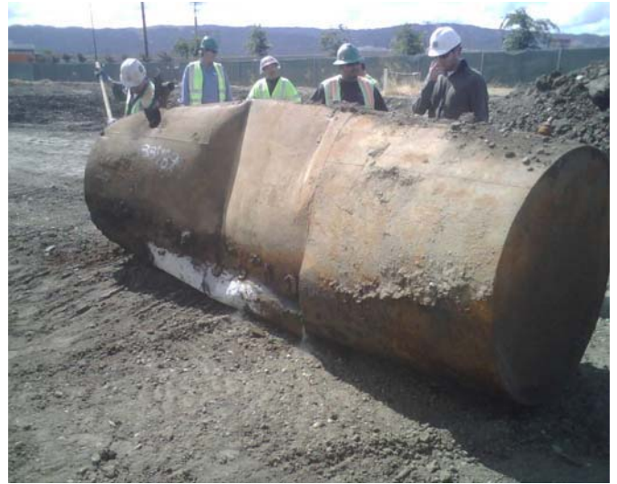
Picture 4 - UST after removal
