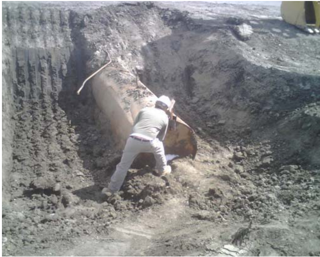
Picture 1 - UST during prior to removal
