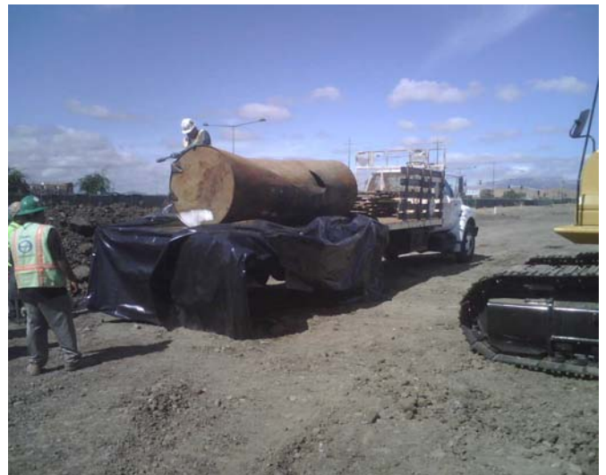
Picture 6 - UST loaded on truck
