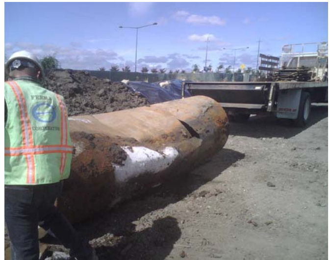
Picture 5 - UST after removal
