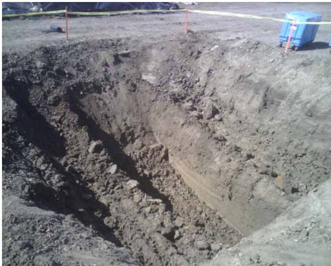
Picture 8 – UST excavation
