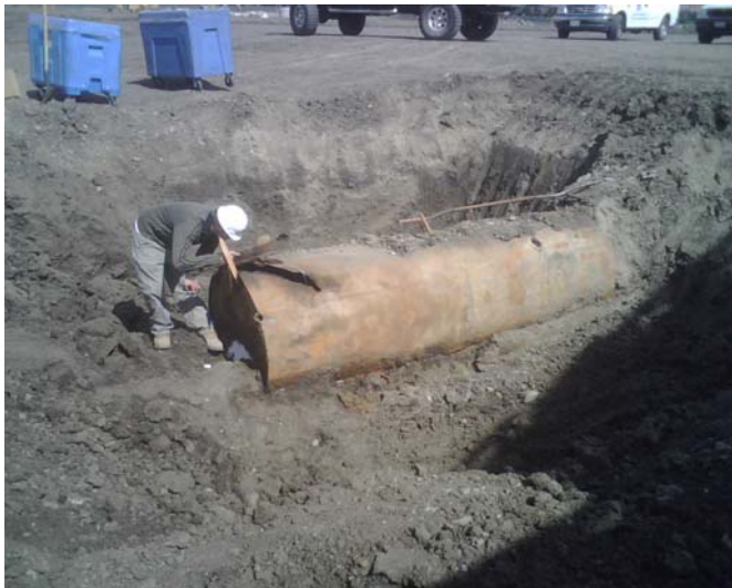
Picture 2 - UST prior to removal
