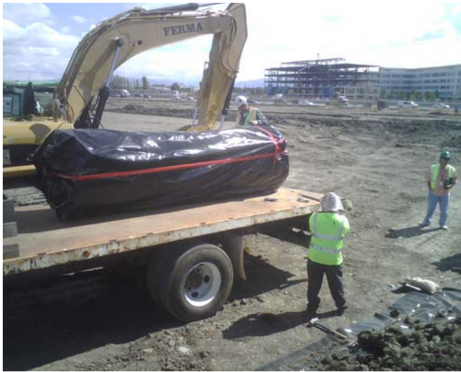
Picture 7 – UST loaded on truck, wrapped in plastic
