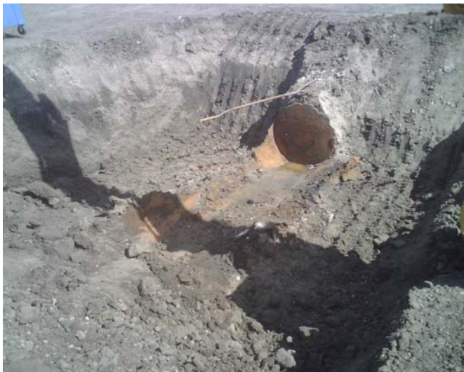
Picture 3 - UST prior to removal
