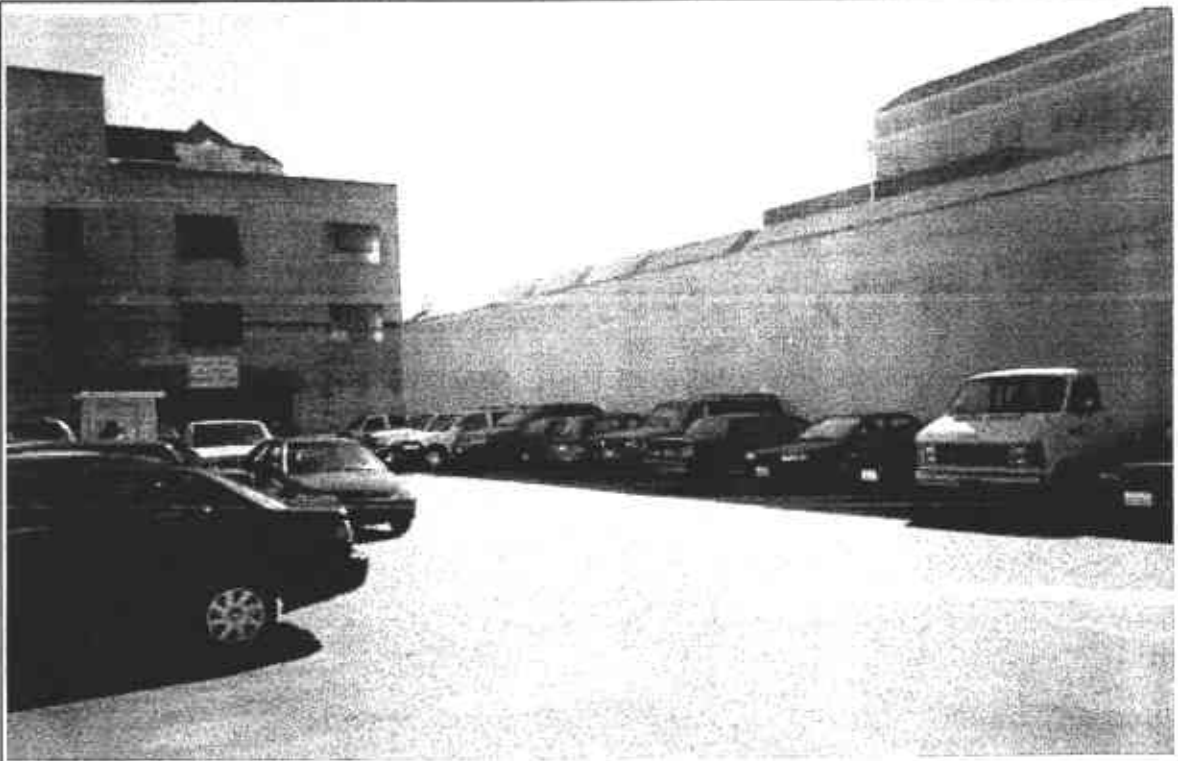
View of 1432 Harrison Street adjacent to the north-northeast of the site.
