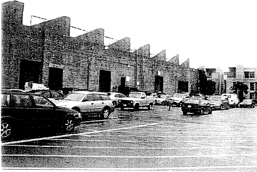
Photo 1. View of east side of Hollis Street building, looking north.
