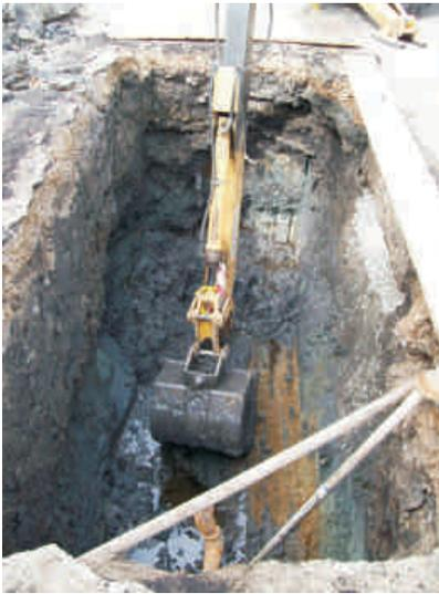
Photo 5. Over-excavation of 1,300 gallon UST cavity.
