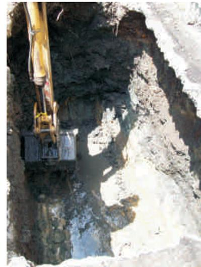
Photo 6. Over-excavation of 425 gallon UST cavity.
