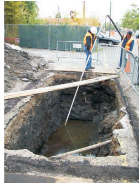
Photo 4. Dewatering UST cavity prior to over-excavation.
