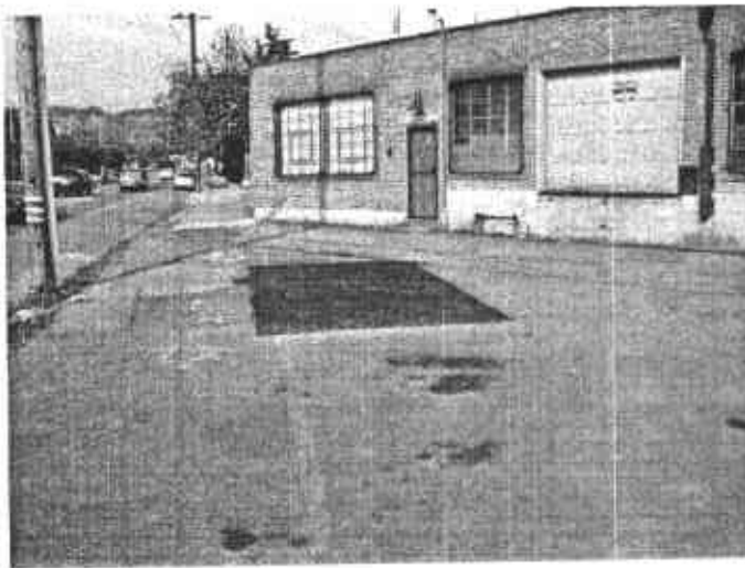
Photo 7. Resurface of former 1,300 gallon UST location.
