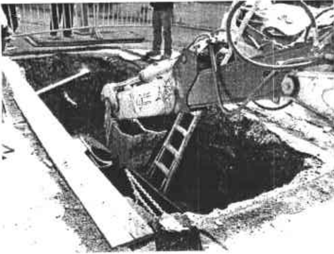
Photo 1. Preparing to remove 1,300 gallon UST.
