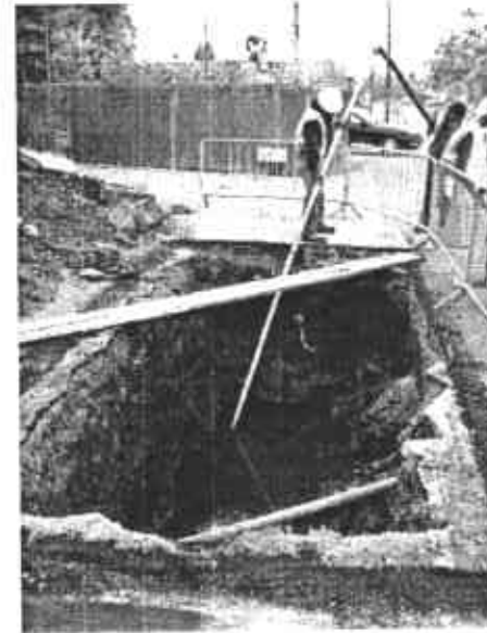
Photo 4. Dewatering UST cavity prior to over-excavation.
