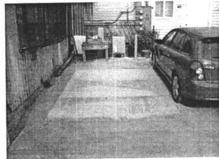
Photo 8. Resurface of former 425 gallon UST location.
