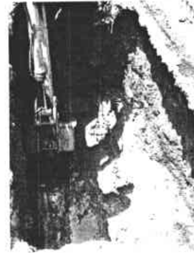
Photo 6. Over-excavation of 425 gallon UST cavity.
