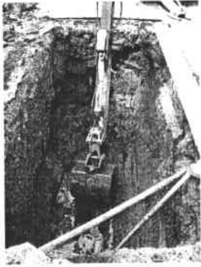
Photo 5. Over-excavation of 1,300 gallon UST cavity.
