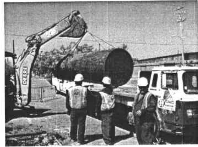
Photo 2. Placing 1,300 gallon UST onto flatbed truck.
