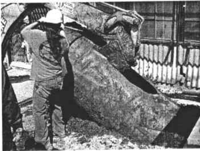
Photo 3. Removing 425 gallon UST.
