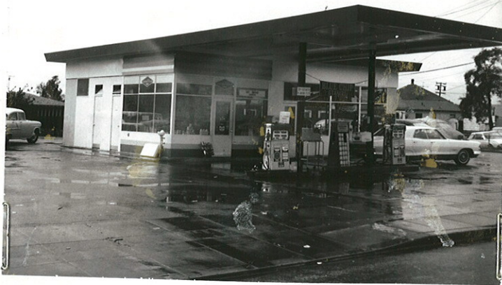
FROM IN FRONT OF STATION, SHOWING PUMP-ISLAND AREA AND SIDE OF BLDG. WHERE RESTROOMS ARE LOCATED
