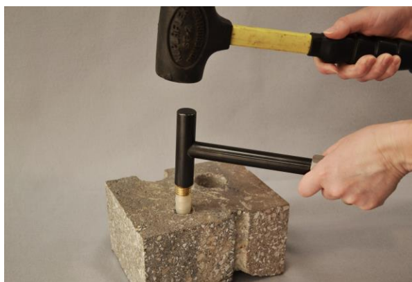
Figure 2. Installing the Vapor Pin™.
