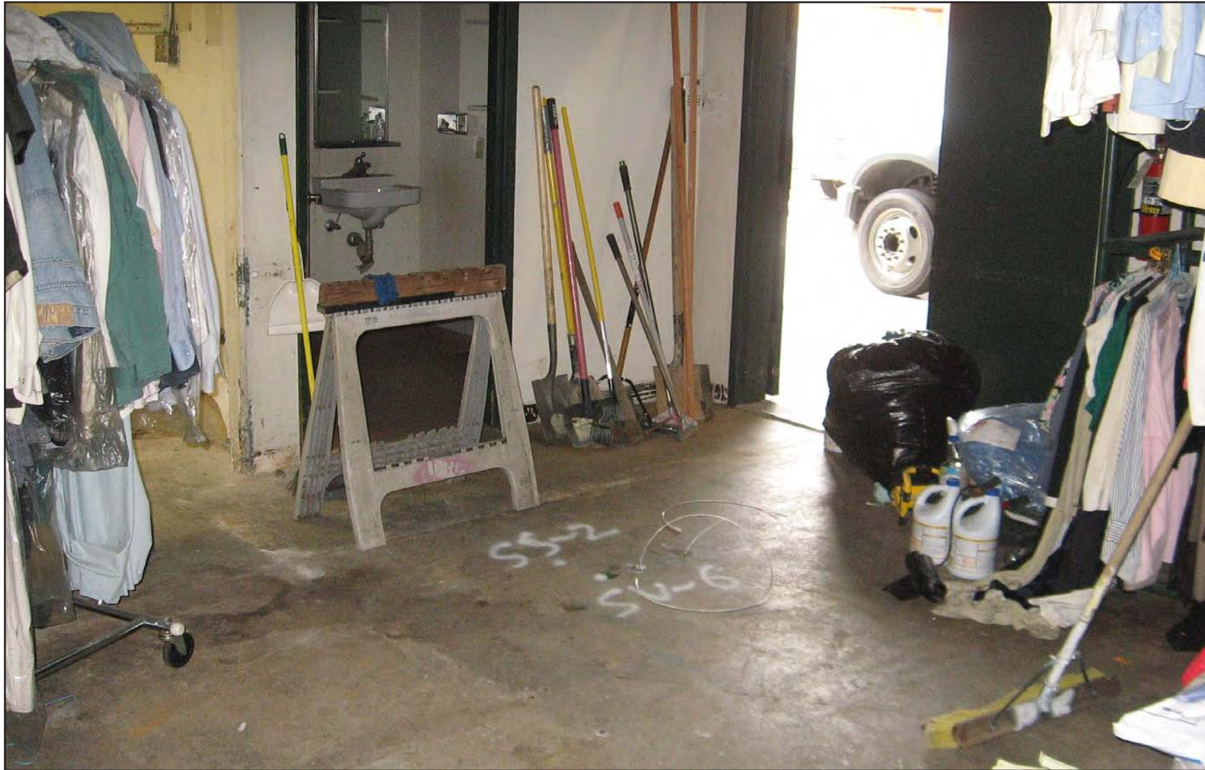
Back of building, east of former dry cleaning machine location.
