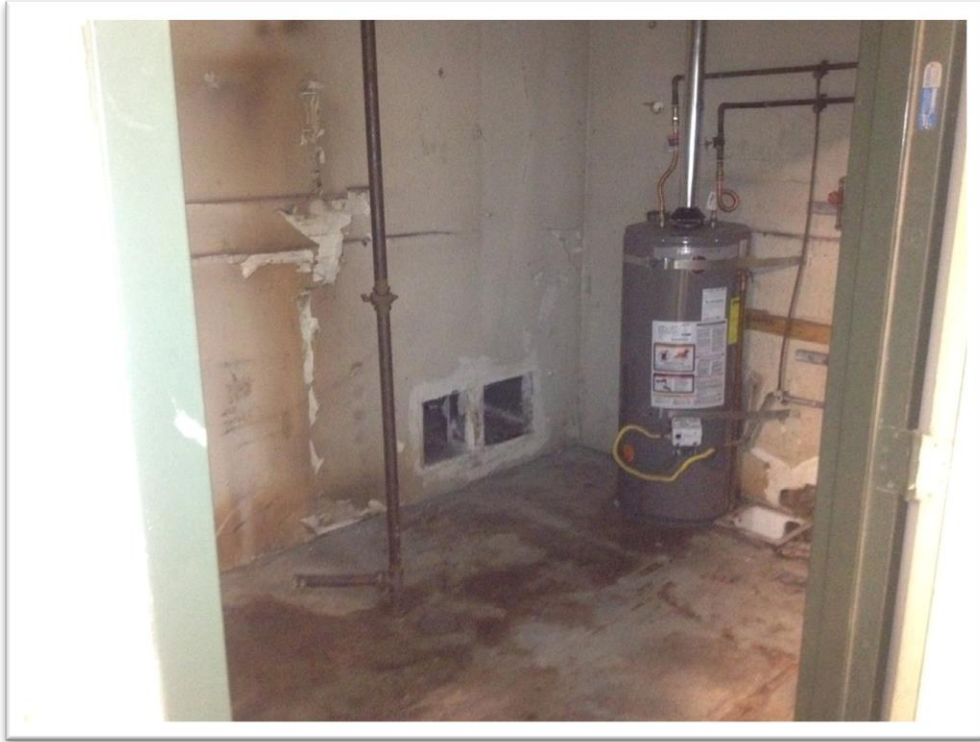
Photo 3. Former Red Hanger Cleaners Boiler Room.
