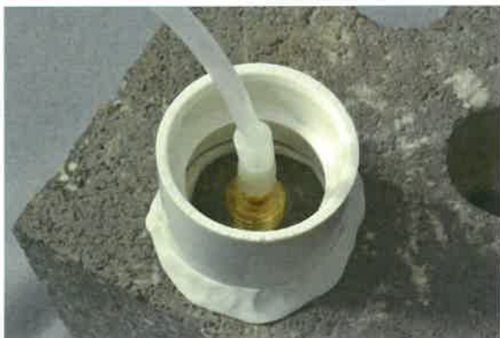
Figure 6. Water dam used for leak detection
