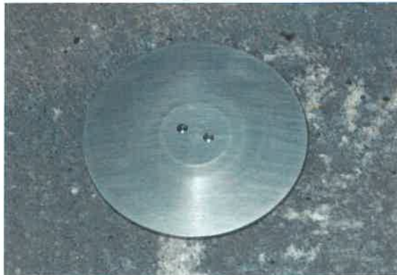
Figure 4. Secure Cover Installed
