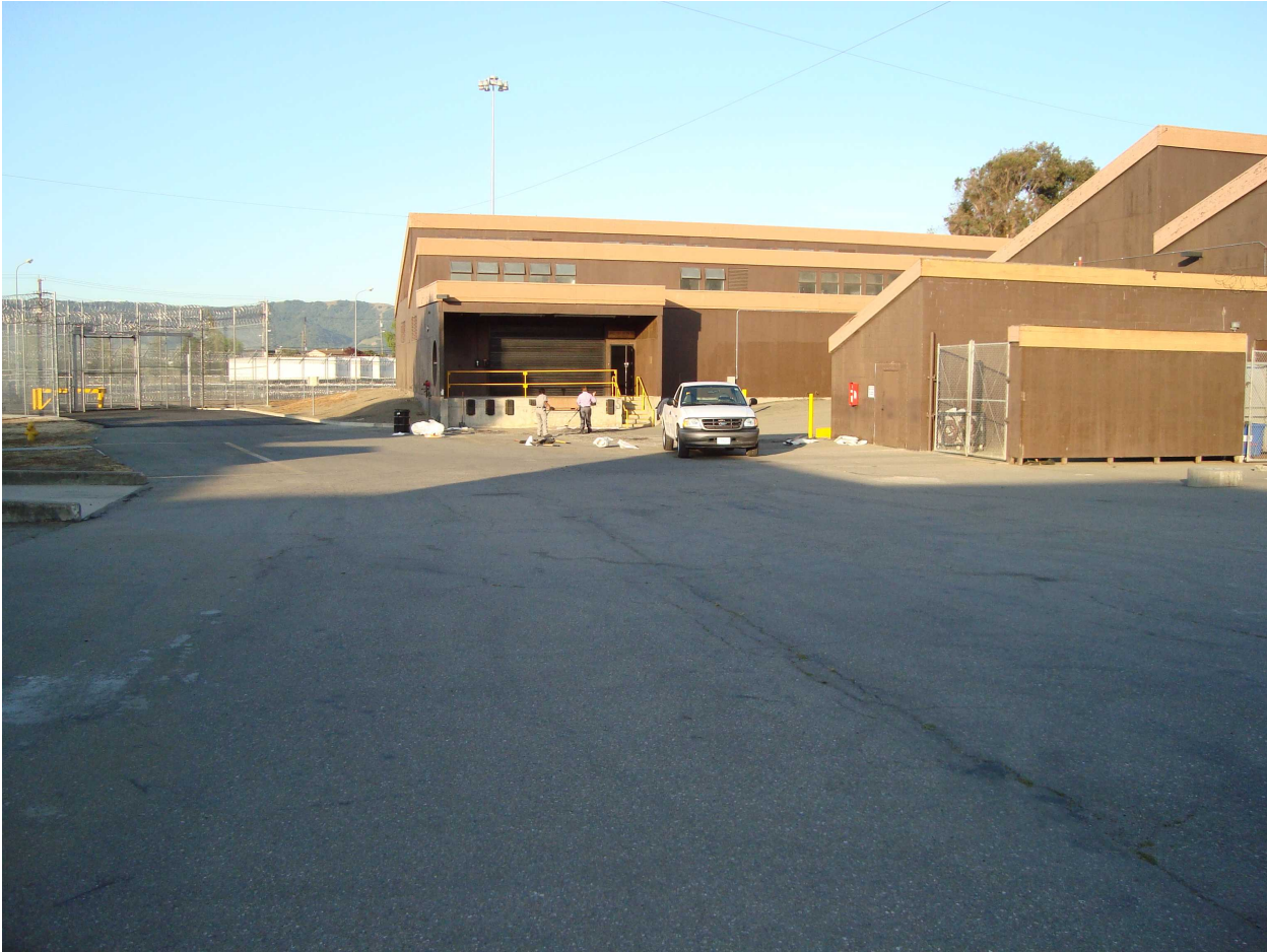
Photo 1: FCI-Dublin Generator Building on right behind chain link gate enclosure. Loading dock well in center, main gate to left. View is to west.
