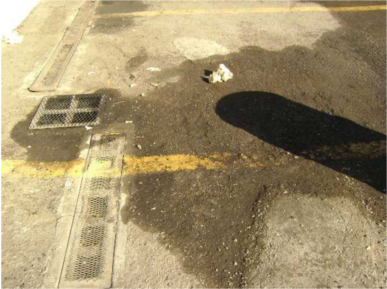
Photo 13: Dock well storm water collection trench and catch basin. View is to the northwest, parallel to dock.
