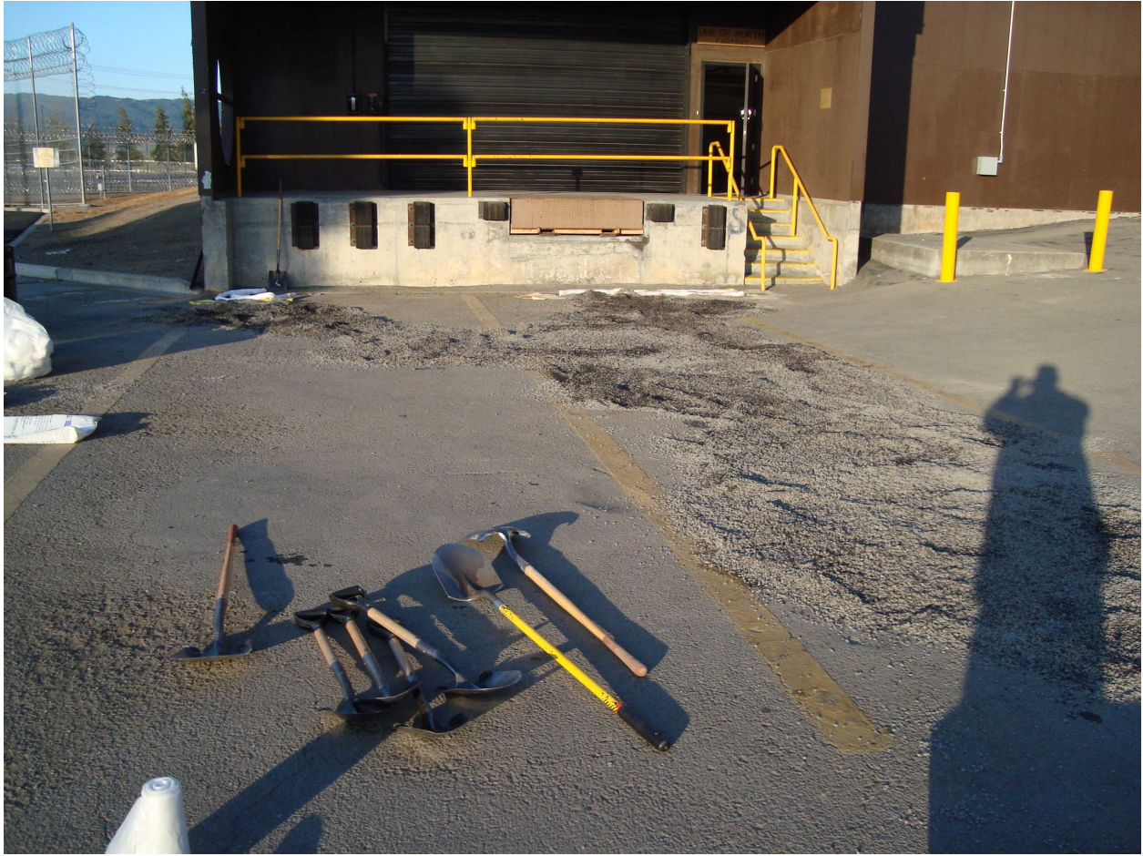
Photo 12: Loading dock and dockwell. View is to the north west.
