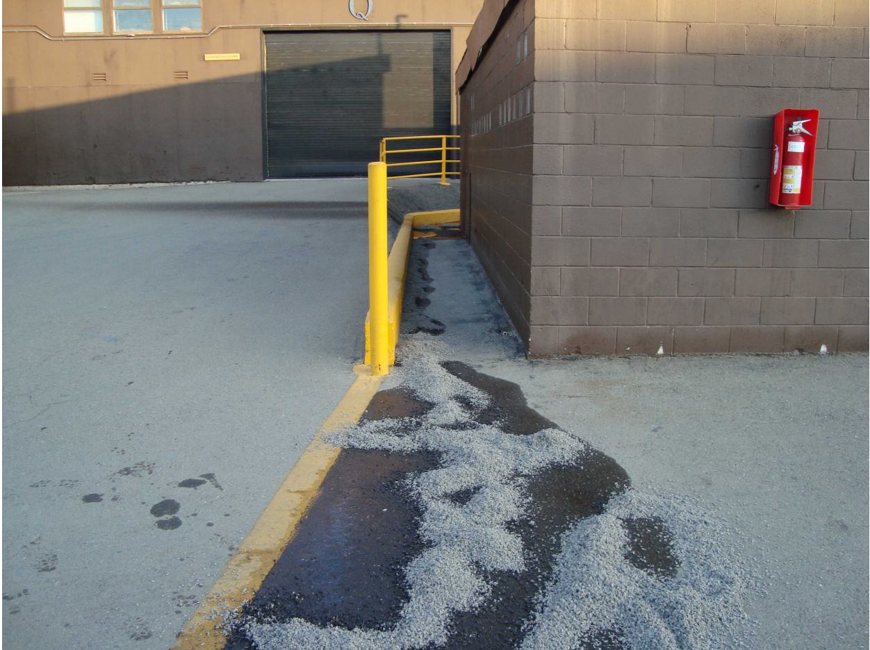
Photo 10: Generator Building, south side. View is to the north.
