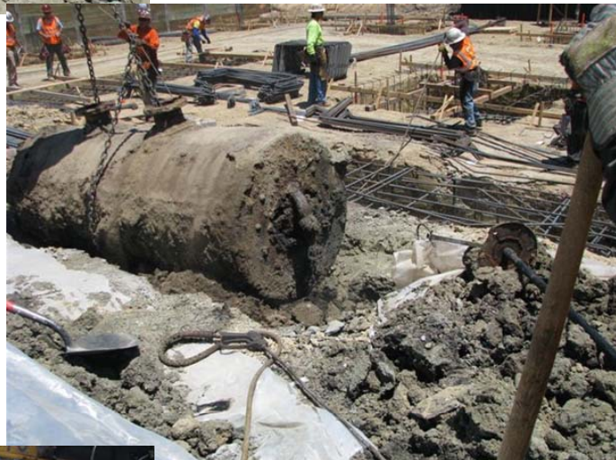
TANK REMOVAL IN PROCESS
