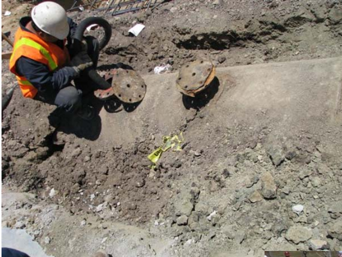
UST READY TO REMOVED FROM EXCAVATION
