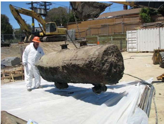
TANK READY TO BE TRANSPORTED FOR DISPOSAL
