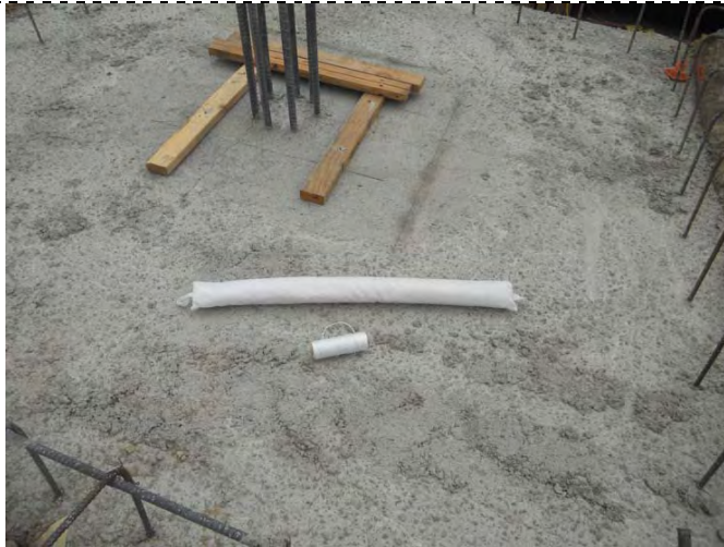
Photograph 1 - Clean Geosorb prior to being lowered into EW-2.
