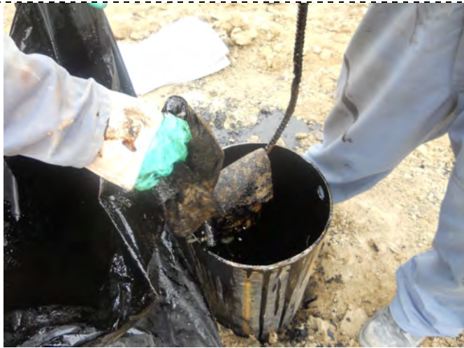
Photograph 7 - Absorbent fabric was used to remove free product prior to abandoning the well.
