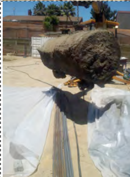
Photograph 6 - Lifting UST from ground and placing onto plastic sheeting.
