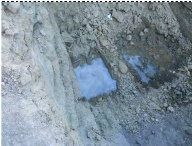
Photograph 15 - Excavation was open for three days, allowing some groundwater to enter.
