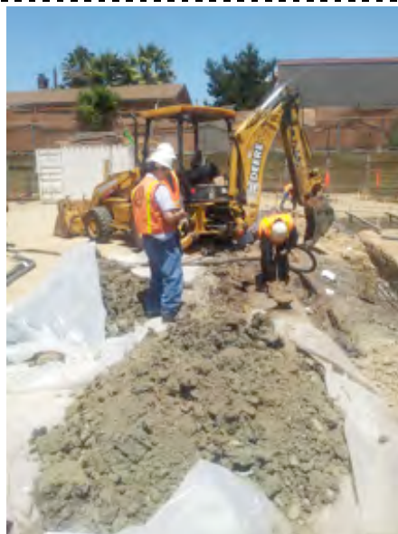
Photograph 3 - Excavated soil was placed on plastic sheeting.
