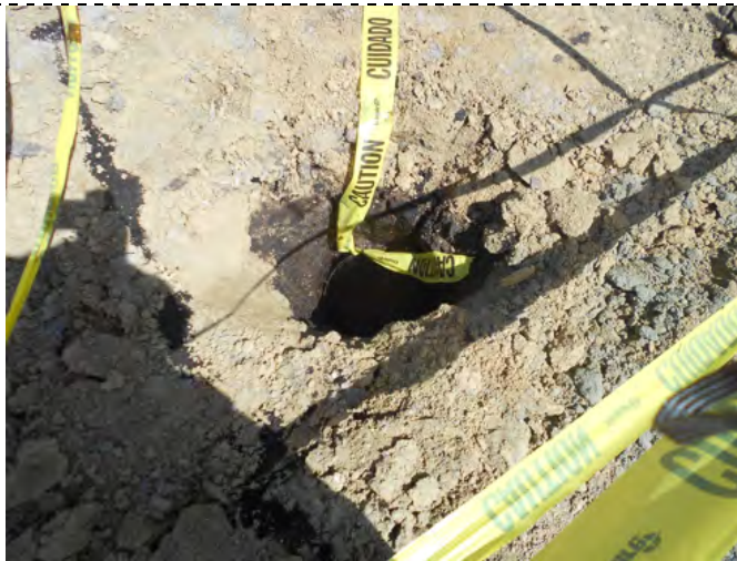
Photograph 1 - 1910 production well the day following discovery.
