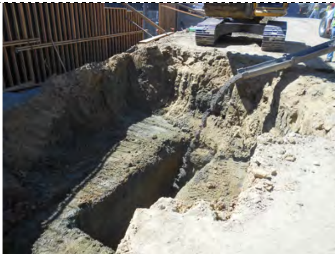
Photograph 23 - The first load of a concrete slurry to secure excavation integrity.
