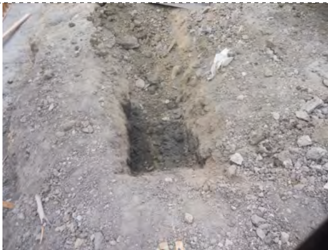
Photograph 11 - Tank pit after removal of UST.
