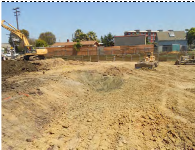
Photograph 3 - Looking north, former UST excavation is in approximate center of photo.
