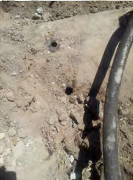
Photograph 5 - Note two holes in top of tank.
