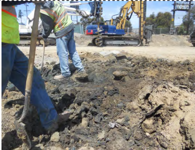
Photograph 1 - Uncovering the top of the UST.
