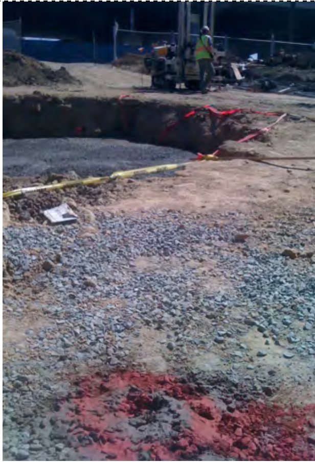
Picture 7 - CPT Rig over MIP-5, taken with MIP-2 in foreground
