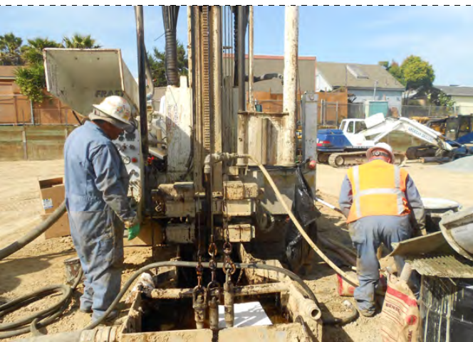
Photograph 11 - Pumping Slurry into the well and water from the well.
