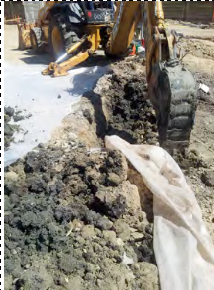
Photograph 2 - Excavating around UST.
