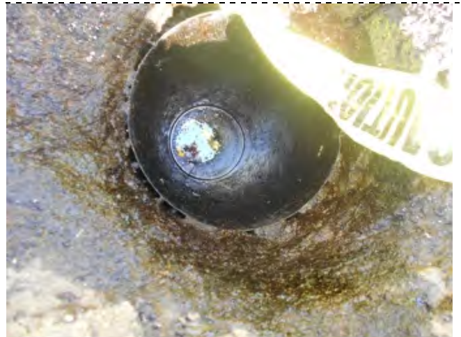
Photograph 2 - Looking down the production well, the day after discovery.
