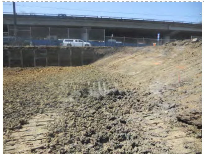
Photograph 6 - Former excavation after filling and covering.
