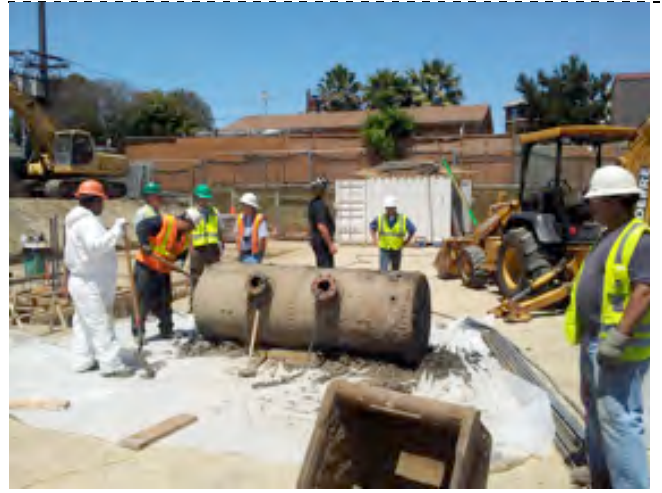
Photograph 8 - Additional photo of UST inspection
