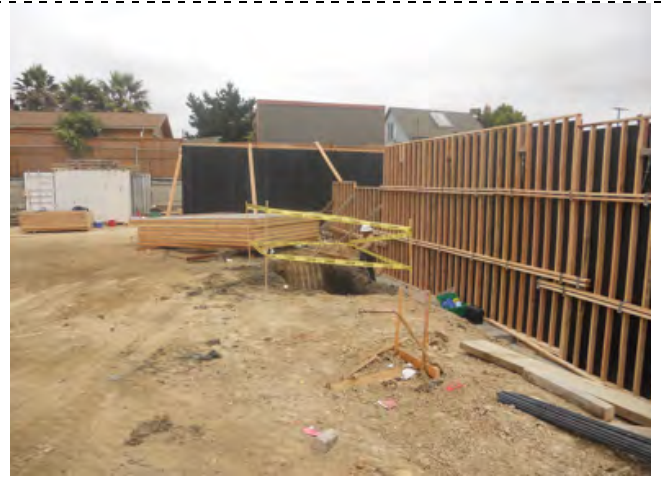
Photograph 14 - Excavation following first day being cordoned off for safety purposes.
