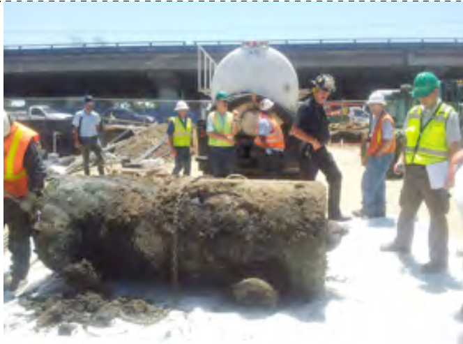
Photograph 7 - Regulators inspecting UST
