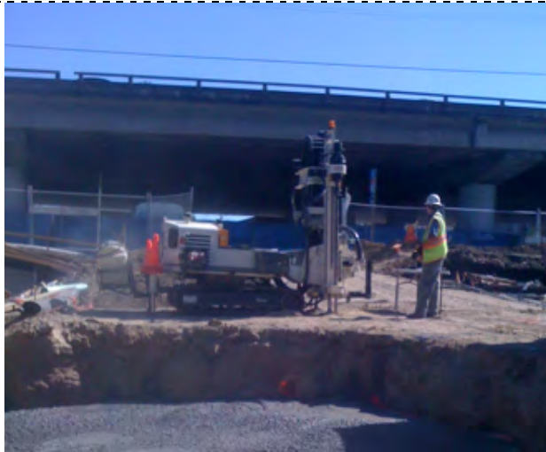
Photograph 1 - CPT Rig over MIP 5, with UST #4 tank pit in foreground.
