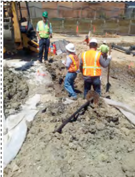
Photograph 10 . Collecting samples from tank pit.
