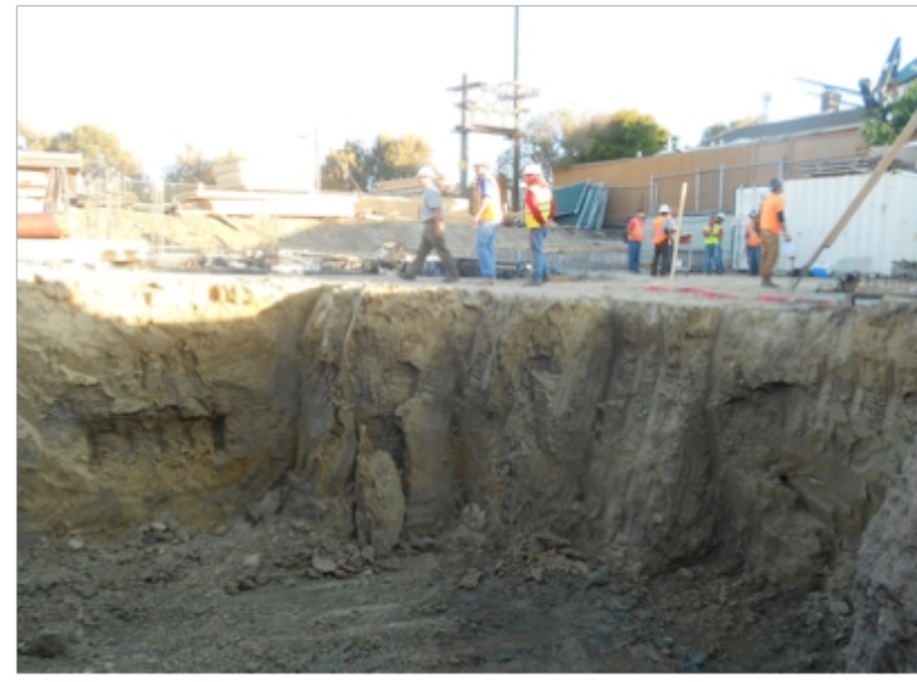
Photo 1 UST 4 - over excavation. Decision was made to stop excavating the width and breadth due to safety concerns. A five-foot deep trench was excavated at the bottom of the excavation, as shown below, in an attempt to remove as much contaminated soil as practical within safety constraints.
