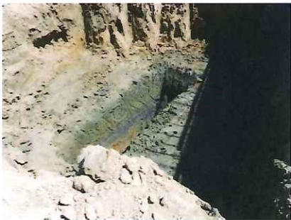
Photo 2 UST 4 - The trench at the bottom of the excavation is five feet deep and as wide as the bucket on the backhoe. The top of the trench is about eight feet below the top of the excavation, which is about five feet below original ground surface. The trench remained open for about 80 minutes while groundwater seeped in at a very slow rate. One liter of water was collected from the bottom of the trench prior to filling the excavation with a concrete slurry due to safety concerns for onsite workers and equipment.
