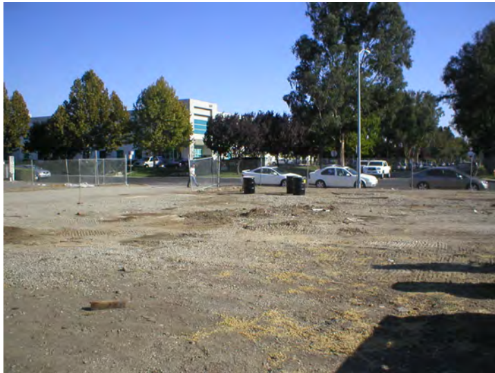
Photo 1. Saddle Tank Area after cleanup
