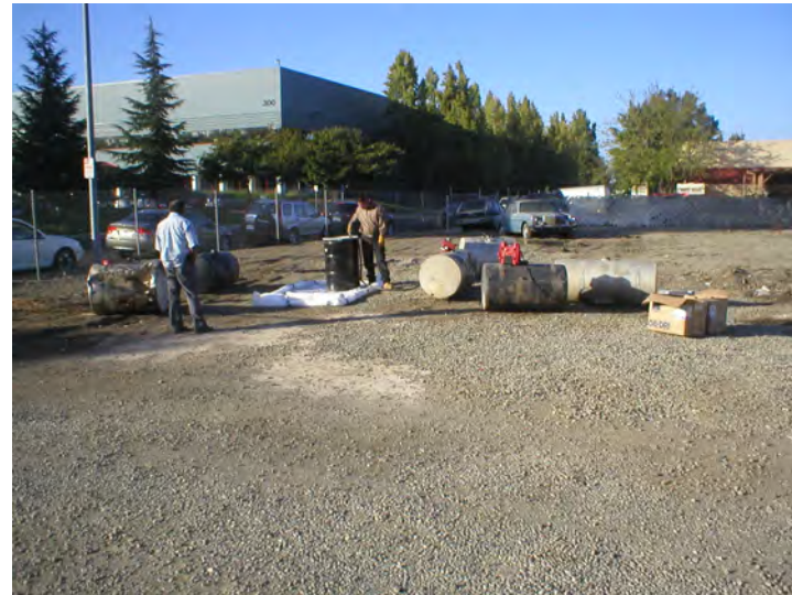
Photo 2. Removal of Diesel Fuel from Saddle Tanks
