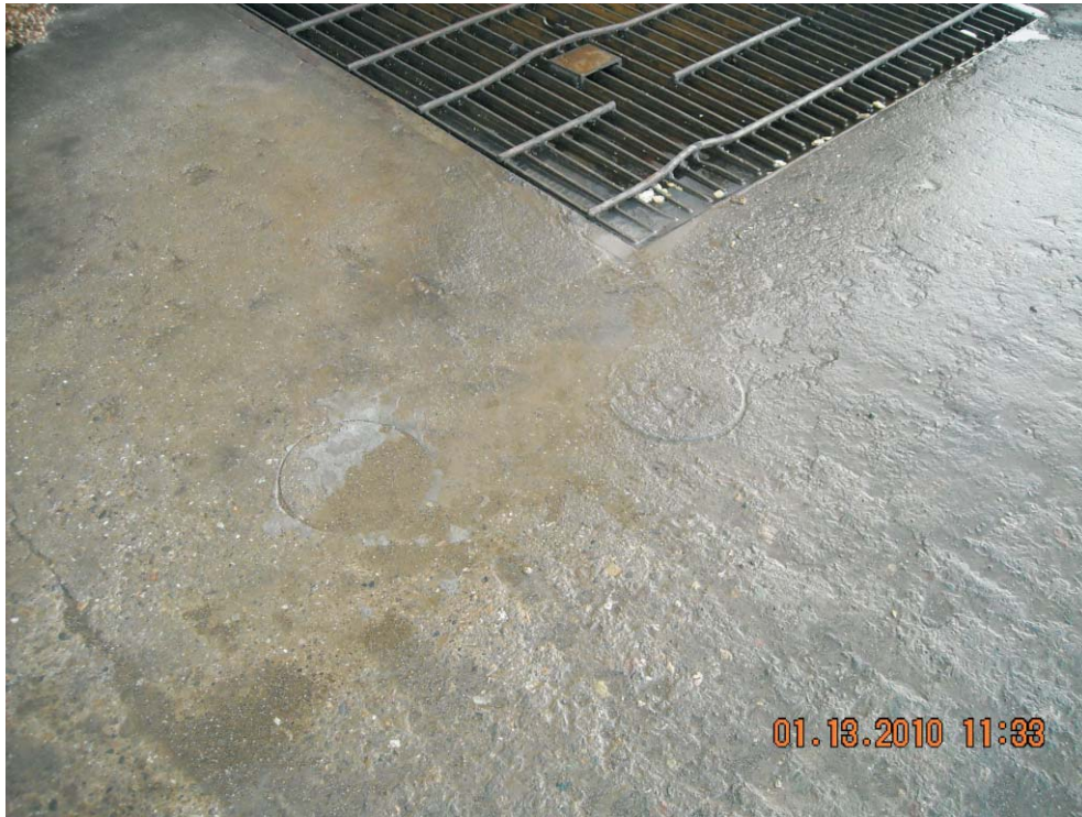
SOIL BORING EB-4 NEAR GREASE TRAP
