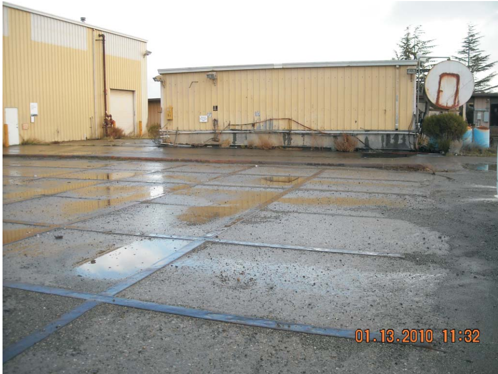
FORMER LUBE SHED LOOKING EAST
