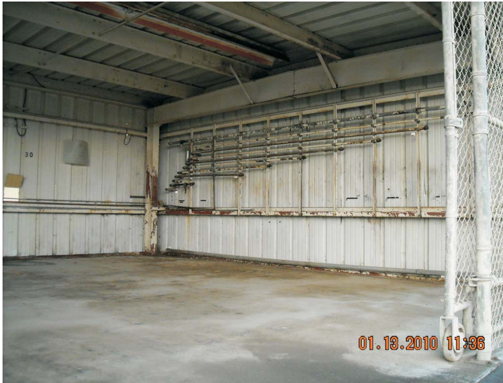
INSIDE THE FORMER LUBE SHED
