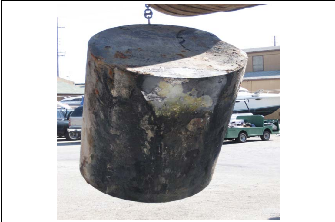
Photograph 5 – Removal of UST #4
