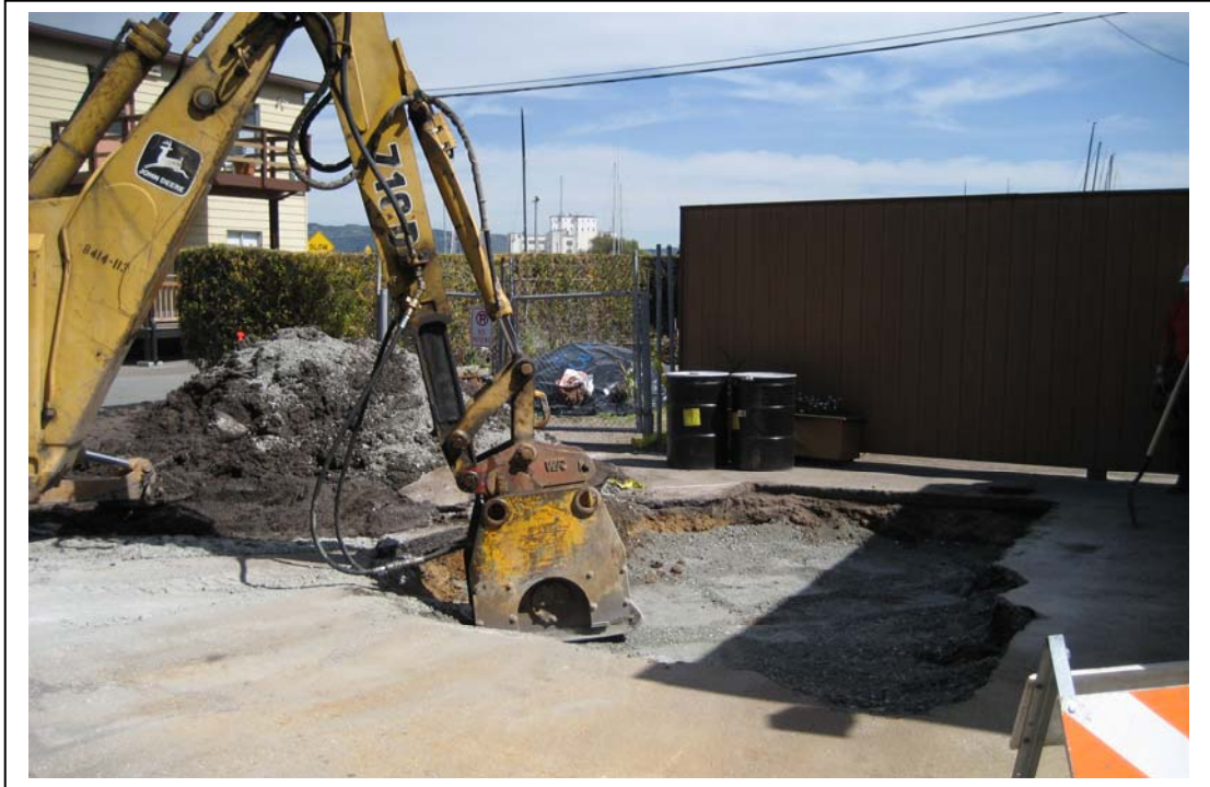
Photograph 11 – Compaction of Backfill Material into UST Excavation
