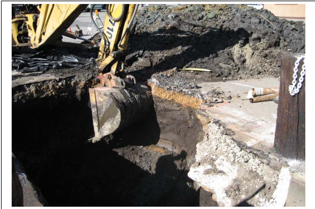
Photograph 6 – Overexcavation of Western Sidewall of UST #2
