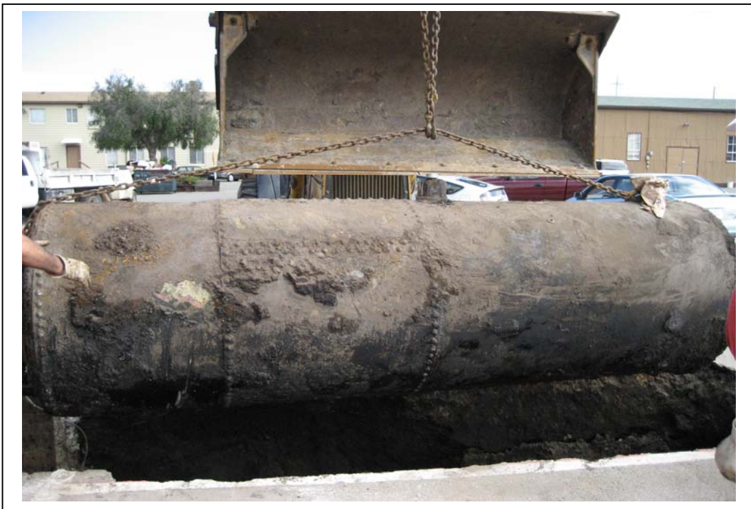
Photograph 2 – Removal of UST #2
