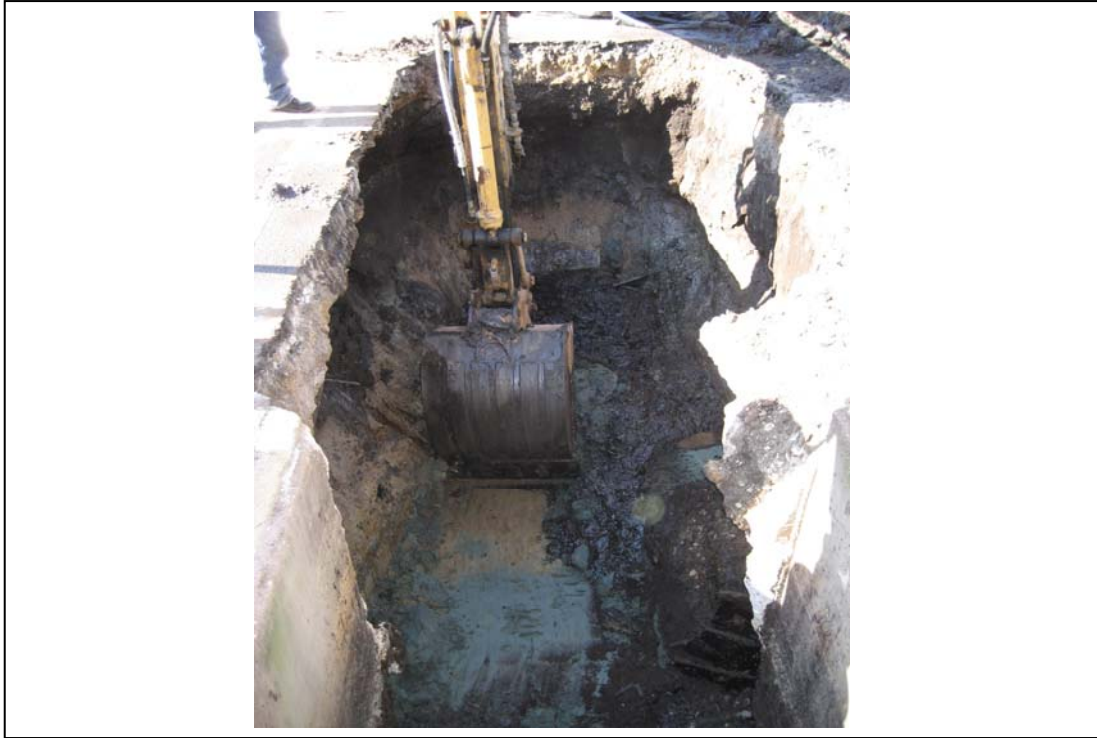
Photograph 7 – Overexcavation of Bottom of UST #2 Excavation
