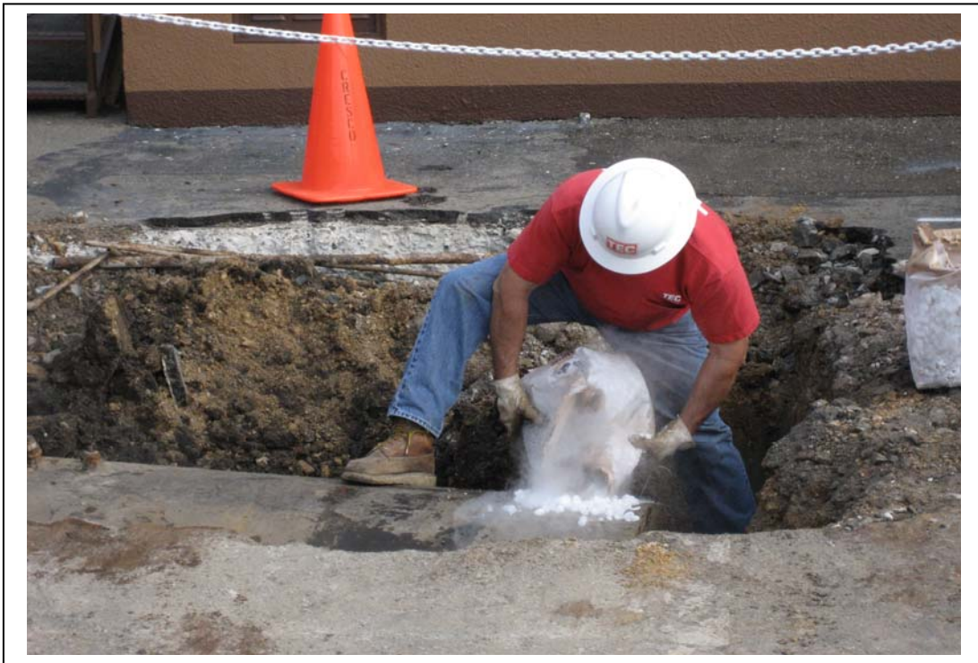
Photograph 1- Dry Ice Placement into USTs
