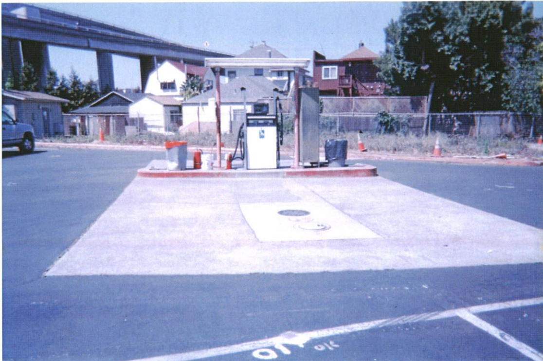
Photo 3: Fuel island, UST, May, 2008.
