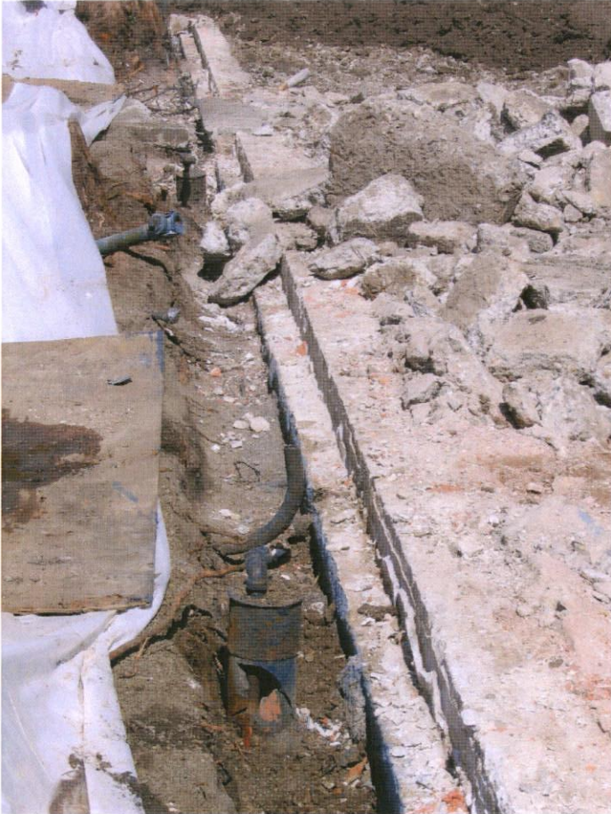
Photo 1: Overview of E and W old piping, slab foundation.
