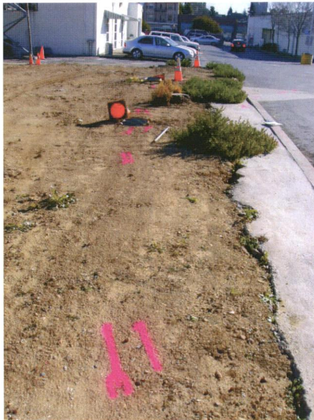
Photo 4: Old building pad, post-demolition.
