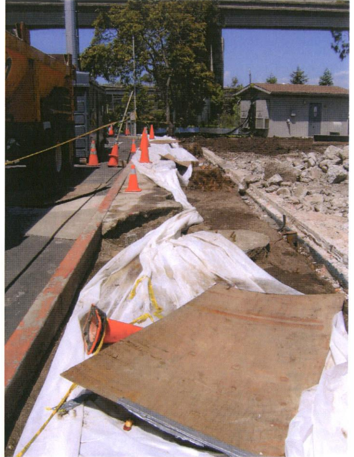
Photo 2: Overview during demolition.
