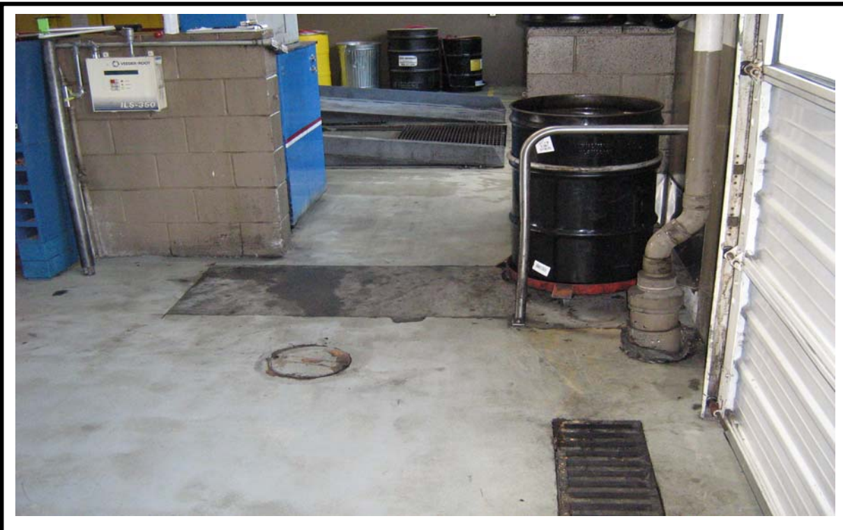
Photograph 3: Restored Former Remote Waste Oil Drain Area Looking West
