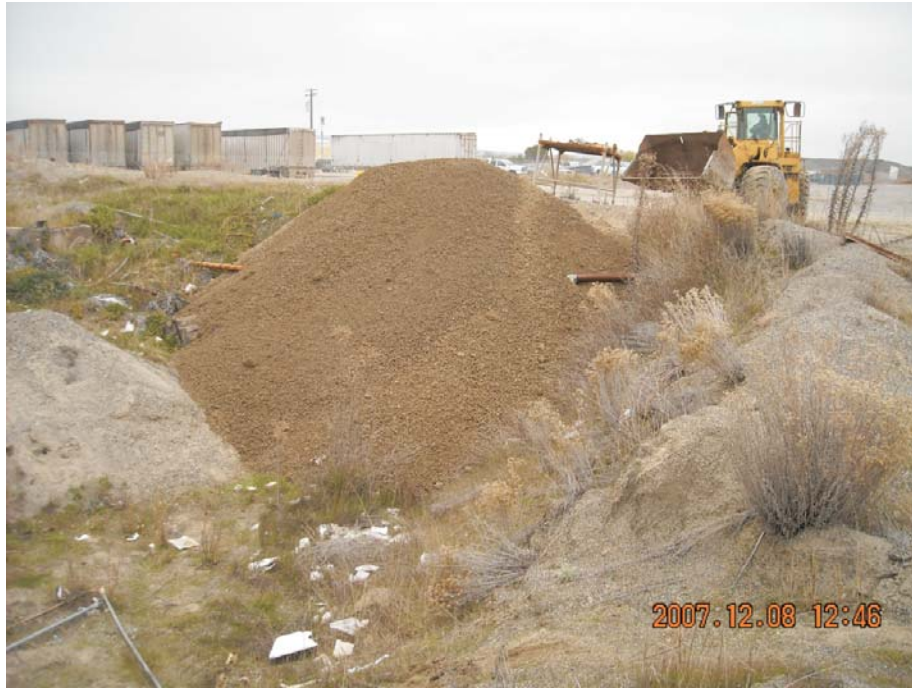
Western Conveyor Entrance Post Abandonment 1
