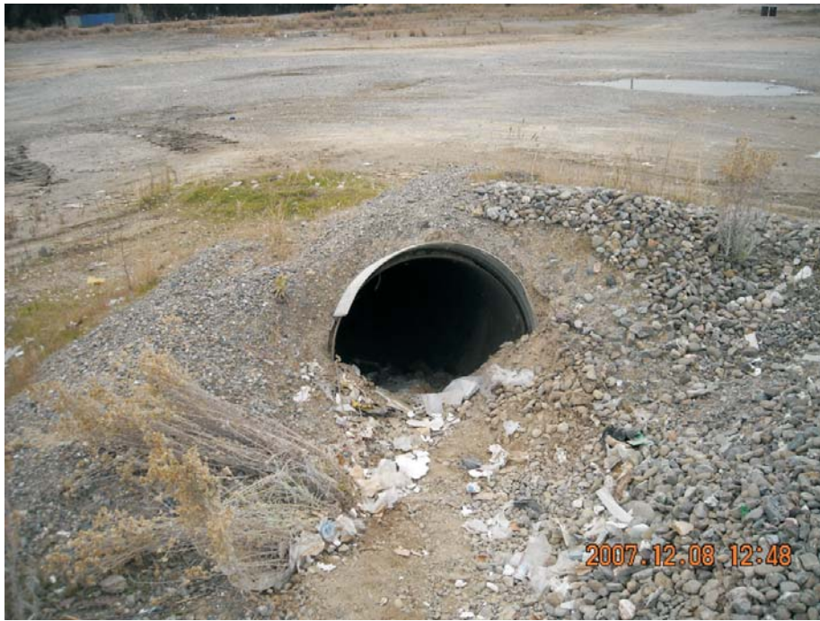
Eastern Entrance to Conveyor Tunnel
