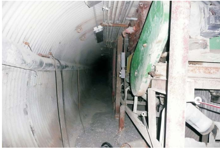
Inside Conveyor Tunnel
