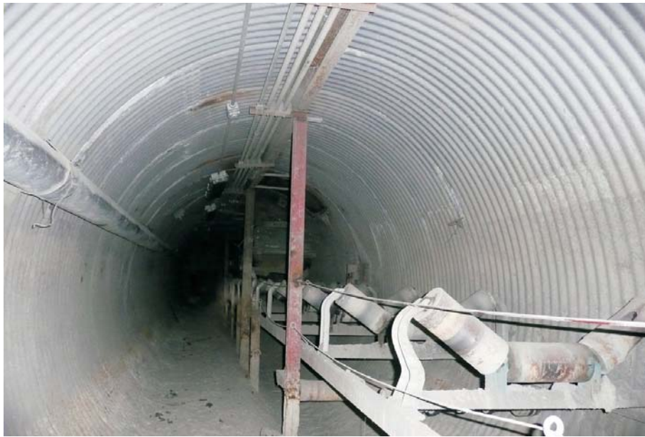
Inside Conveyor Tunnel
