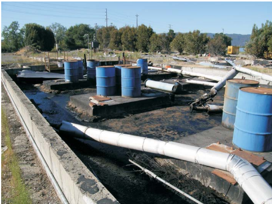
Drums in Containment Structure 1
