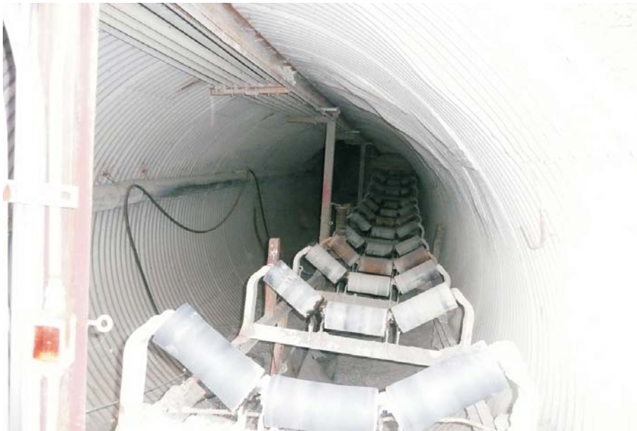
Inside Conveyor Tunnel
